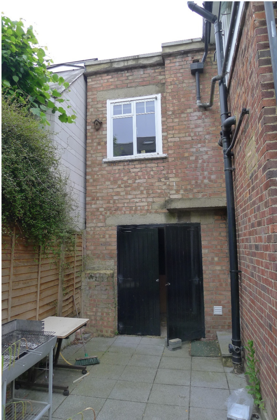
View of rear elevation of the garage from the garden
