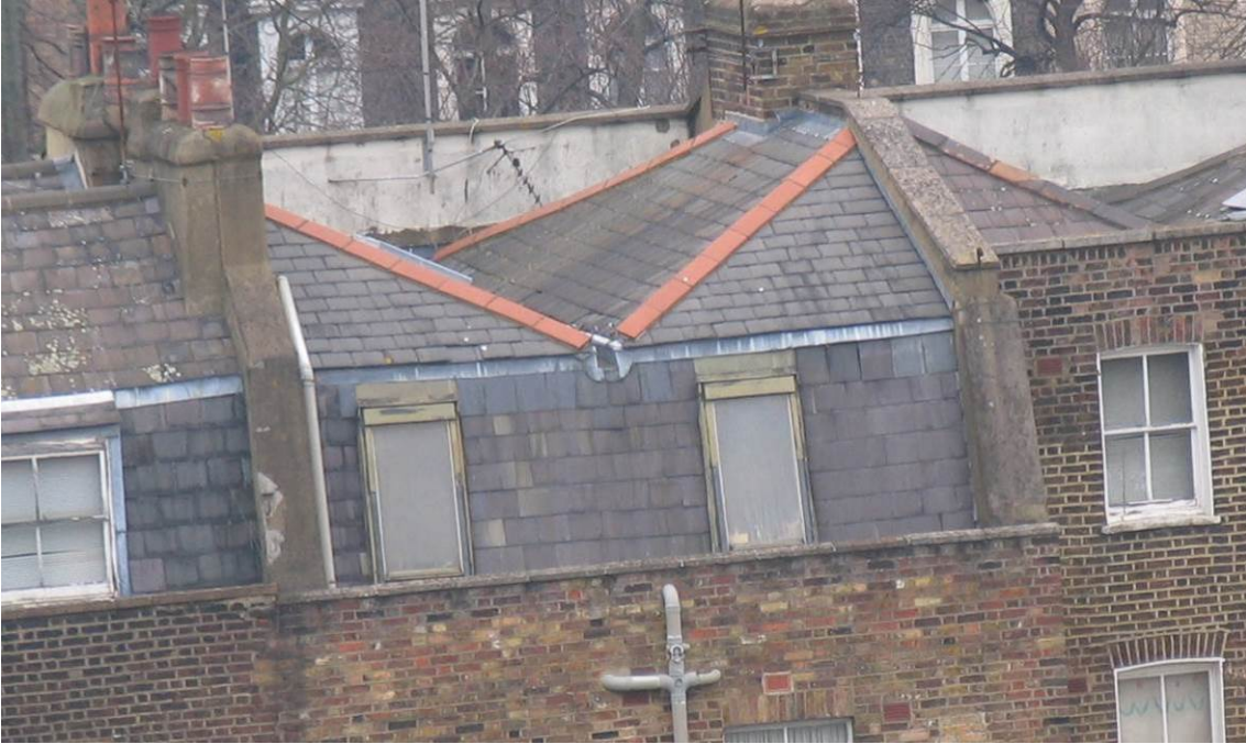
Roof viewed from rear
