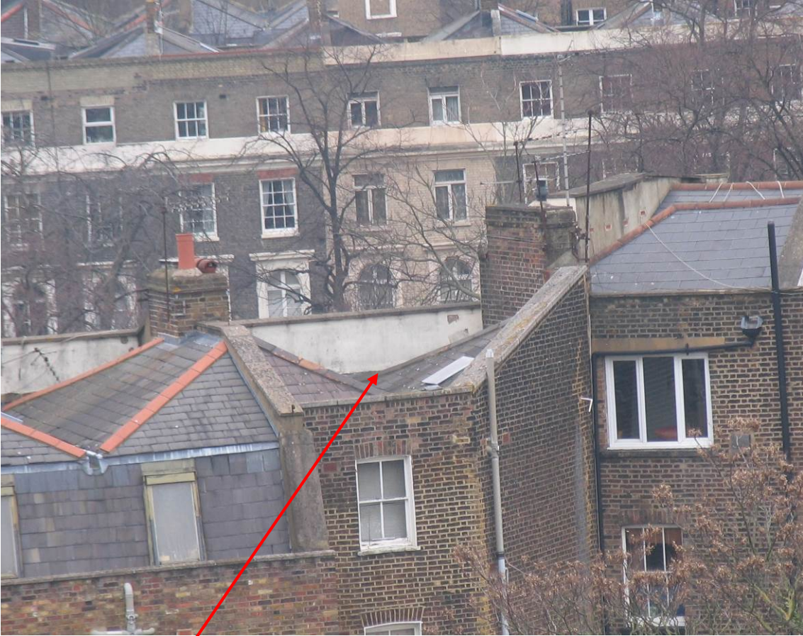
Roof viewed from rear
