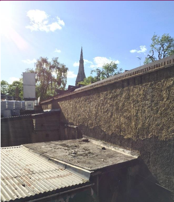
View of Rear Looking North West
