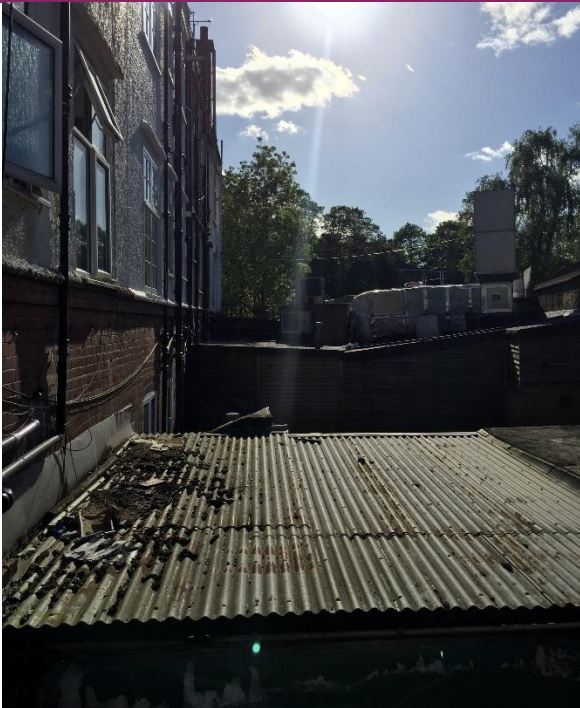
Existing Roof of the Outbuildings, Looking West
