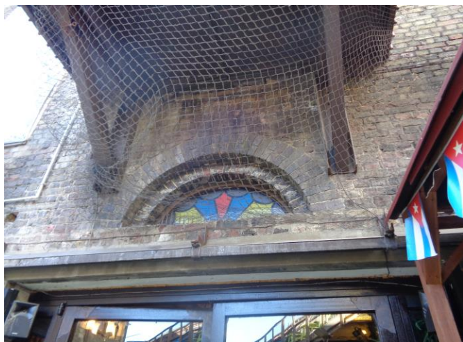
Fig.6 Fanlight window, east elevation
