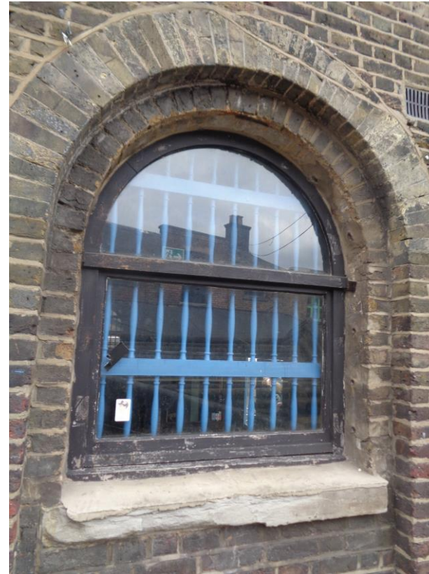
Fig.4 Timber window, ground floor, north elevation
