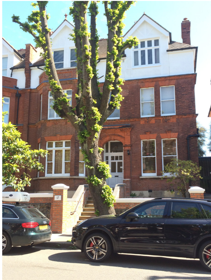
Fig.2. Existing front Elevation of 17 Chesterford Gardens. Photo taken from across the street on Chesterfors Gardens.
