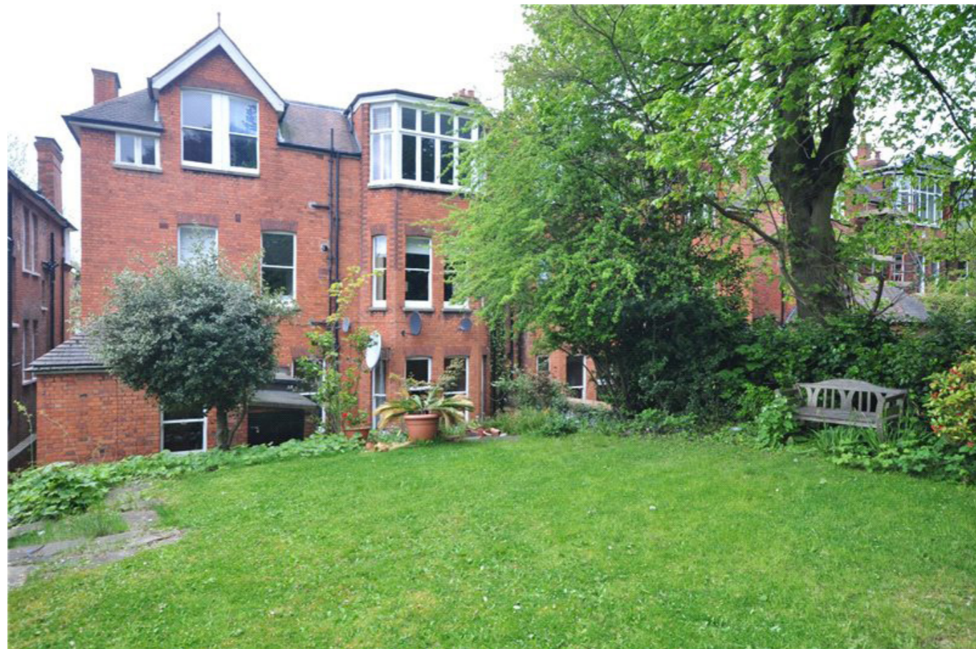
Fig. 3. Existing rear elevation. Photo taken from existing private garden looking back to house. Photographed supplied by the ground floor flat.
