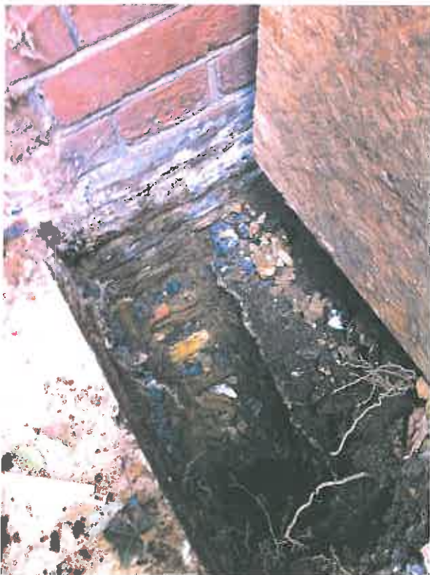
TP2(2015) – View into pit showing brick corbel and underlying rubble foundation
