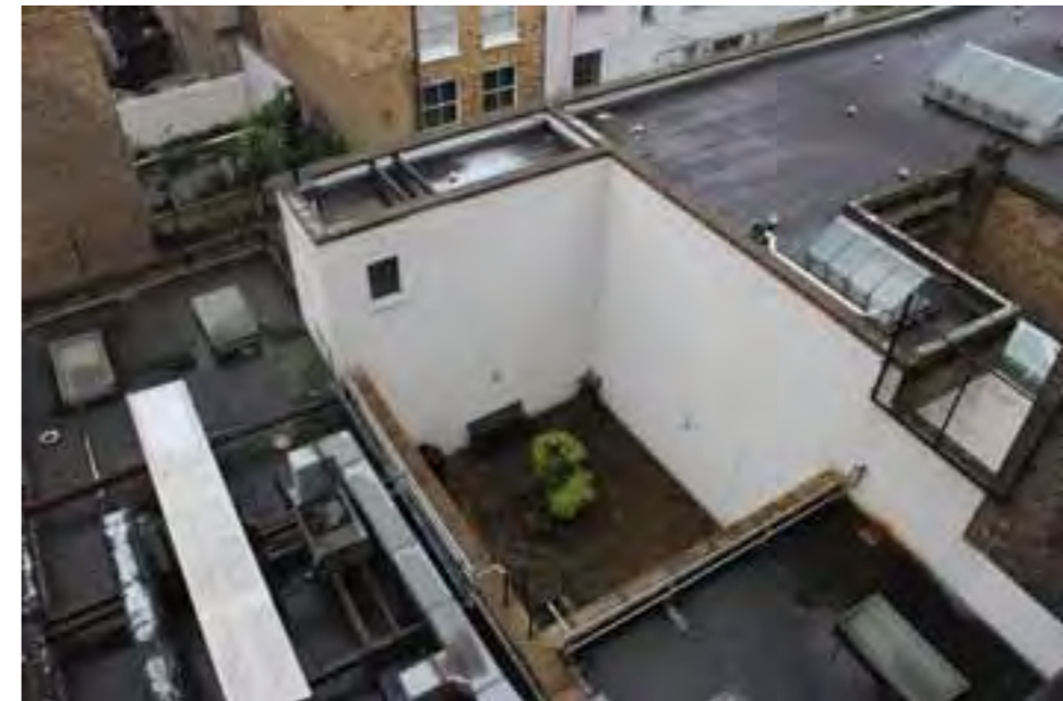
FIG 28. REAR EXTENSIONS TO NOS.14 AND 15
