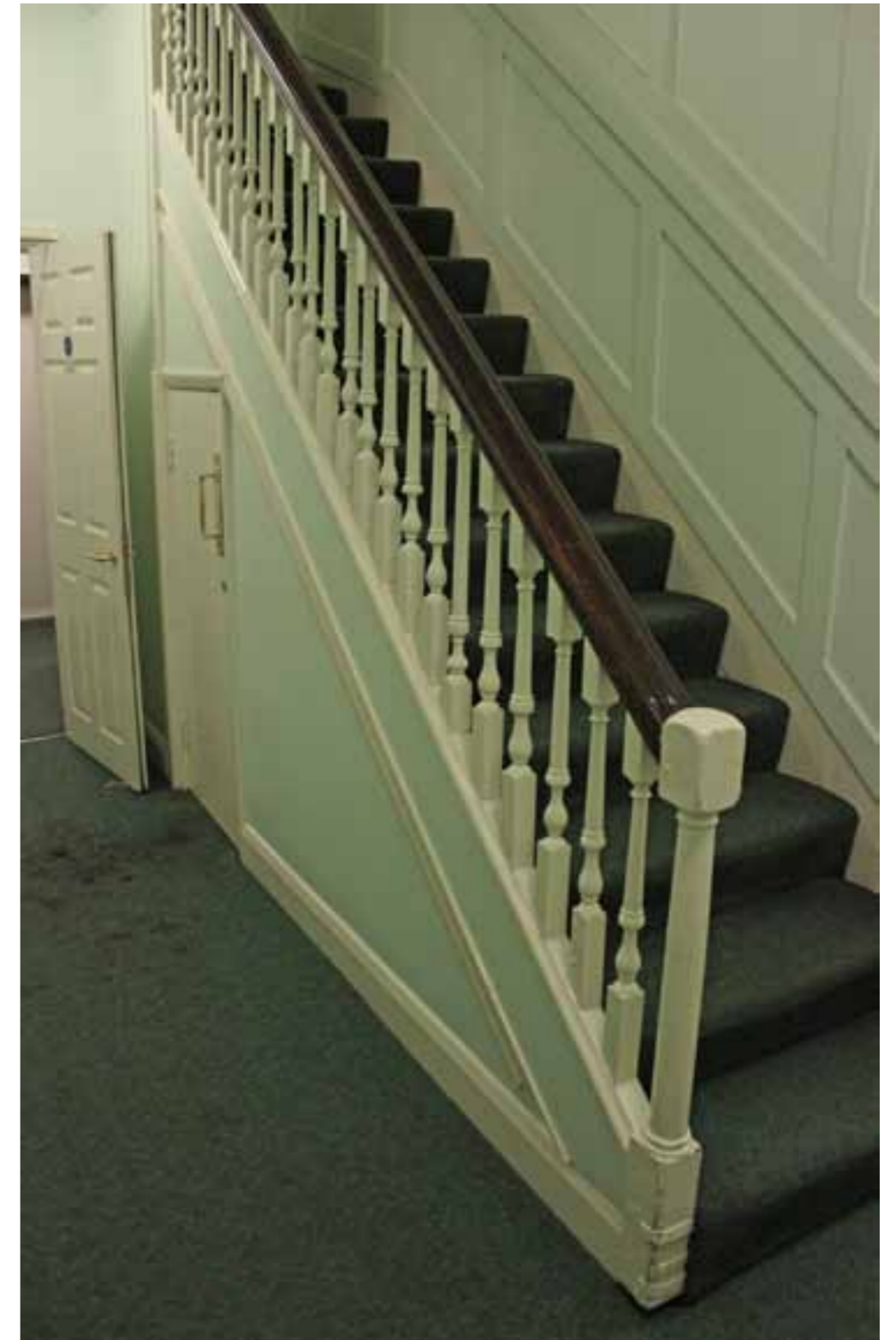
FIG 39. BASEMENT STAIR AND PANELLING AT NO.14
