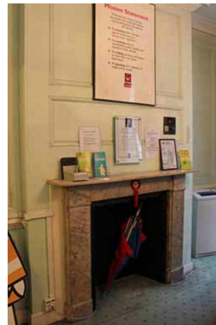
FIG 43. GROUND FRONT ROOM FIREPLACE AT NO.14
