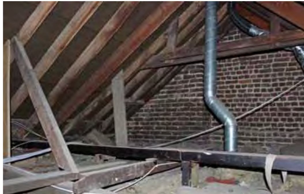
FIG 35. MAIN ROOF VOID AND PARTY WALL
