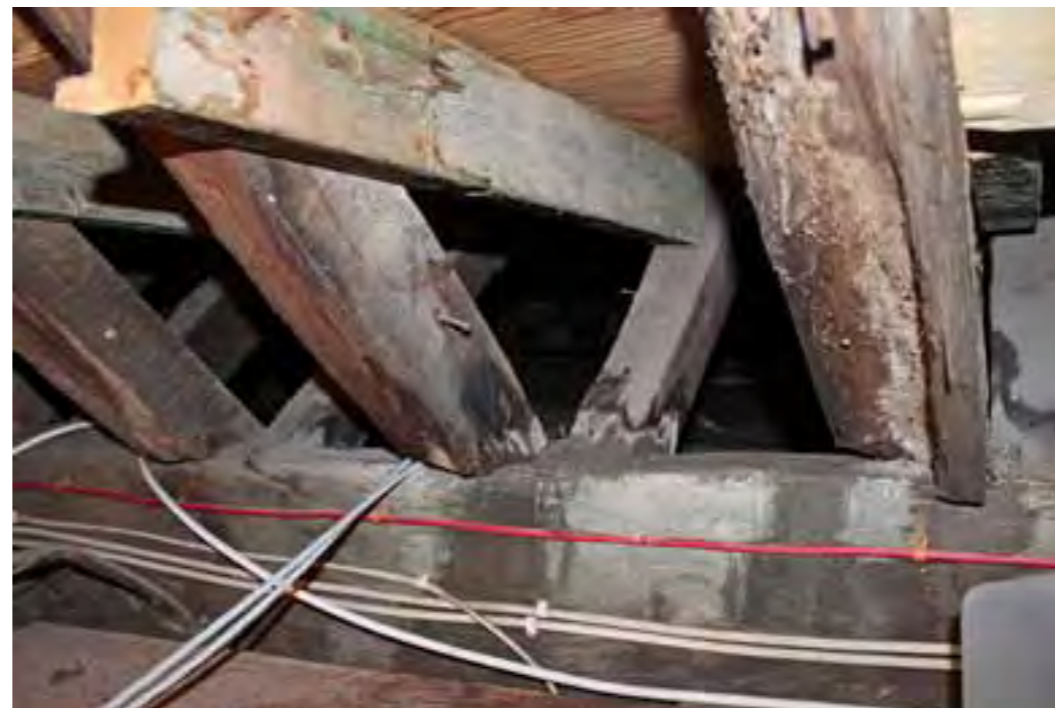
FIG 36. MAIN ROOF VOID AND VALLEY GUTTER
