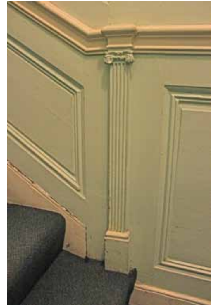
FIG 53. SECOND FLOOR STAIR PANELLING AT NO.14
