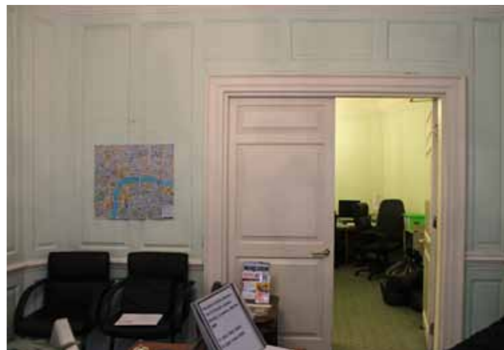
FIG 40. GROUND FLOOR FRONT ROOM AND PANELLING AT NO.14
