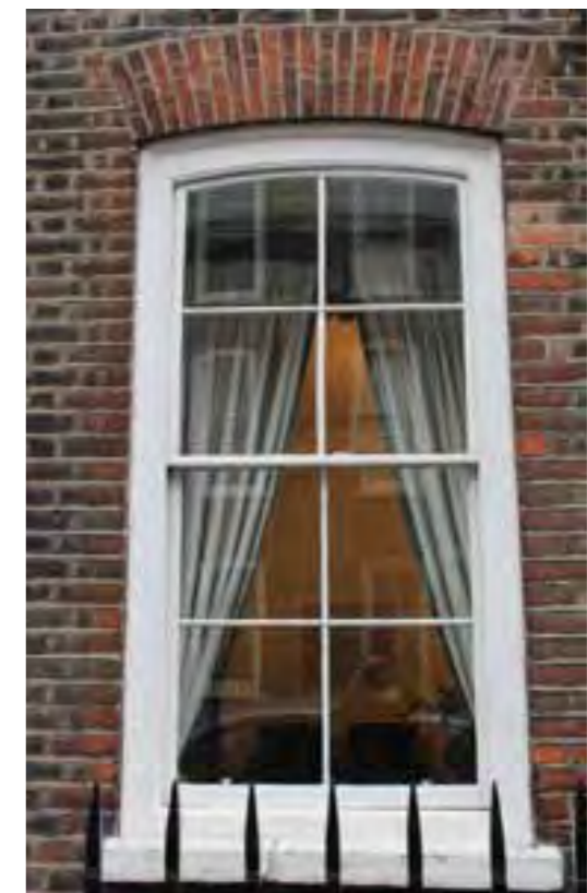
FIG 25. FRONT GROUND FLOOR WINDOW TO NO.14
