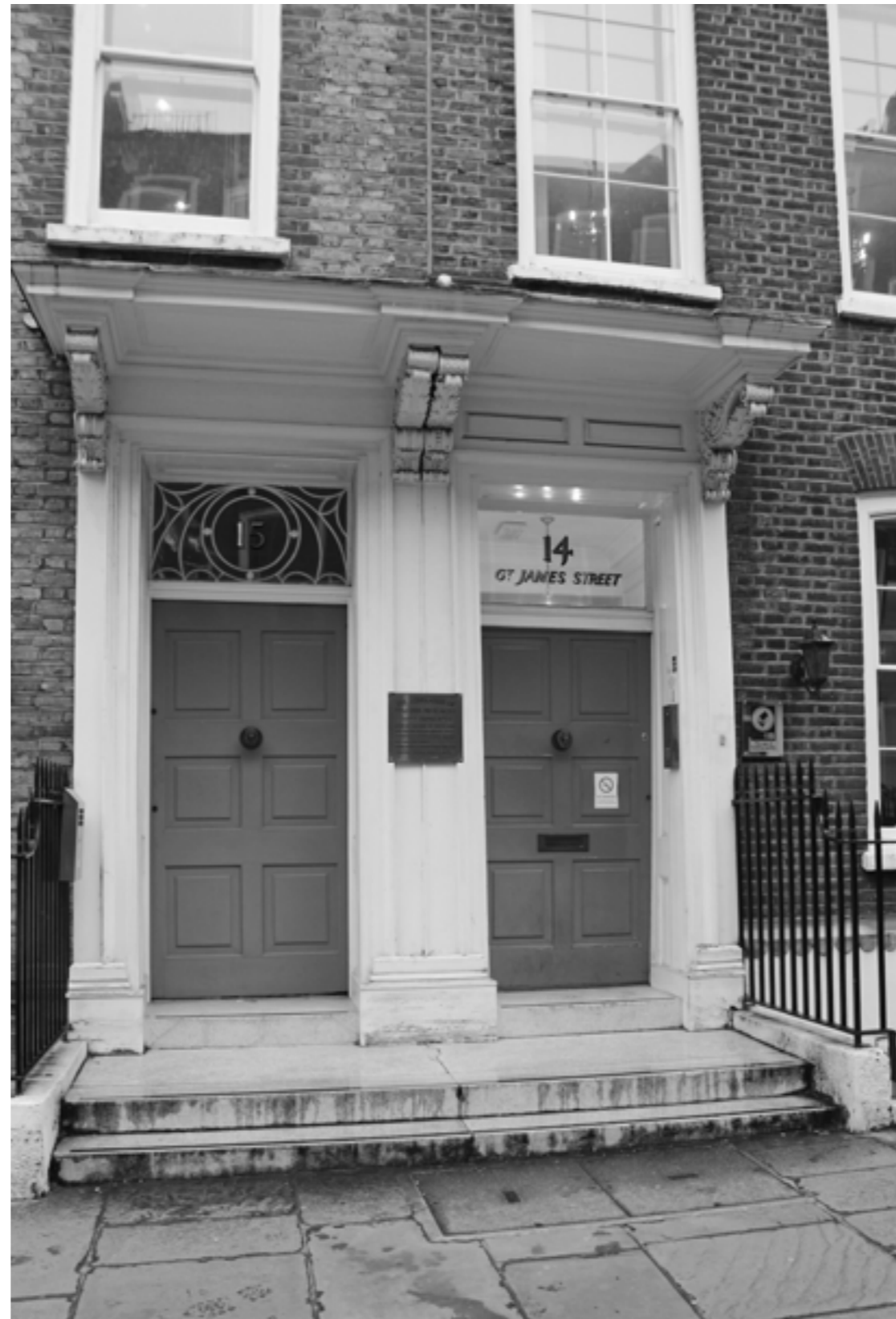
FIG 23. 2013 PHOTOGRAPH OF FRONT DOORCASES TO NOS. 14 AND 15 (REFER TO FIG.19 1960 PHOTOGRAPH)
