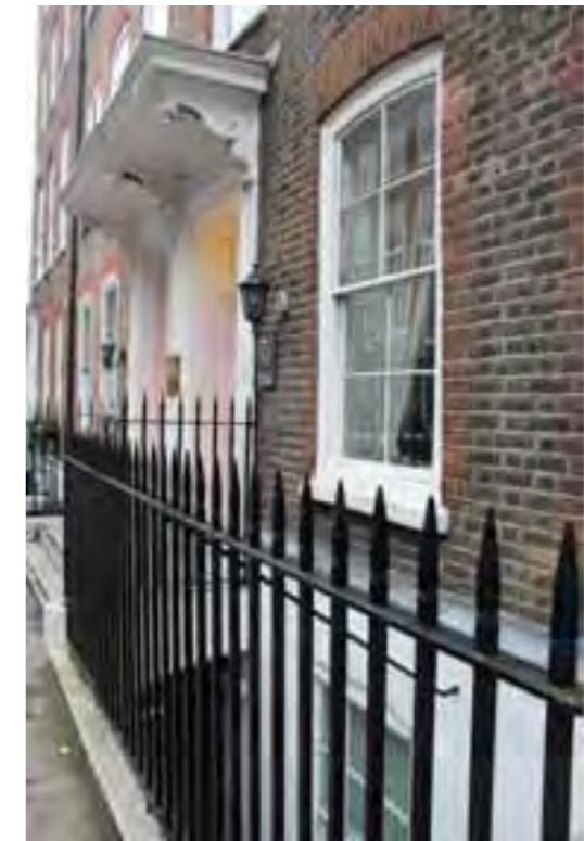
FIG 24. STREET FRONTAGE TO NO.14
