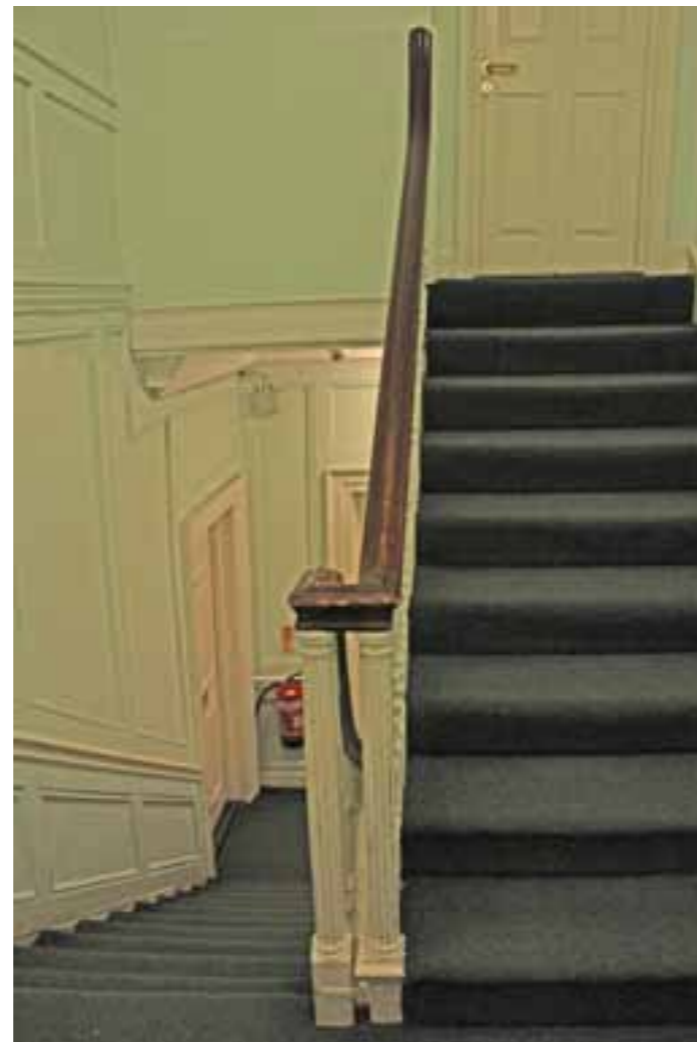
FIG 56. THIRD FLOOR STAIR AND HALF LANDING AT NO.14
