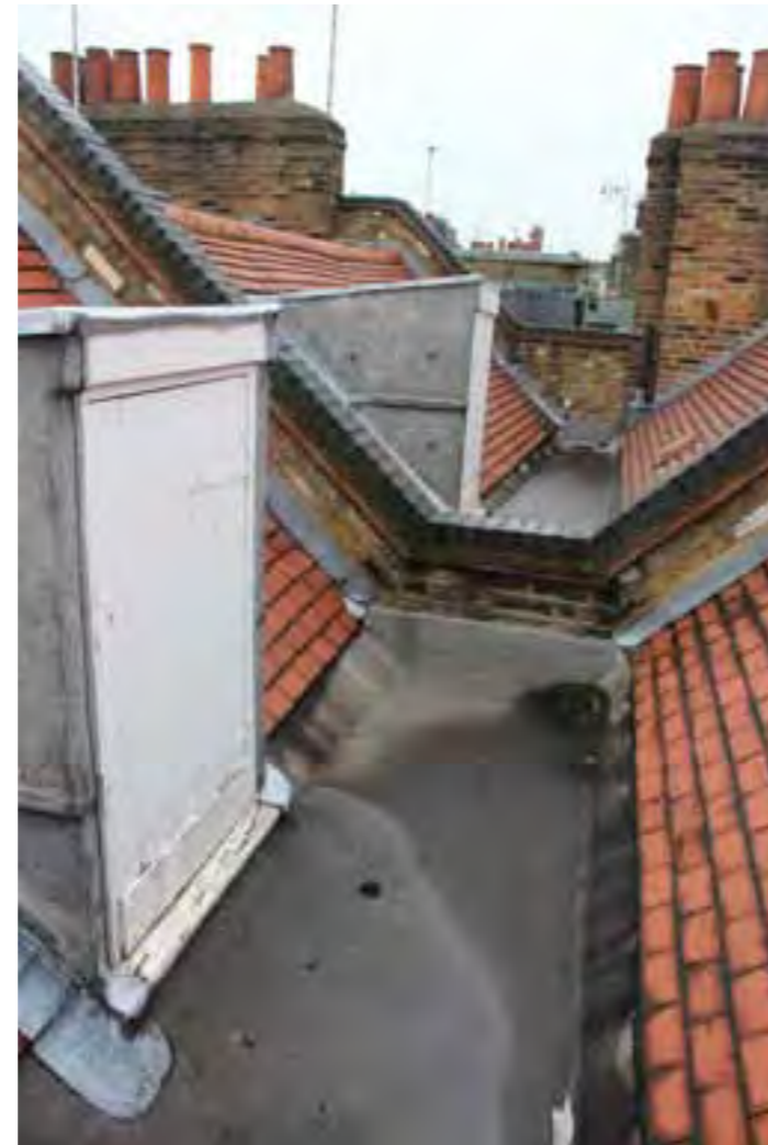
FIG 30. MAIN ROOF AND VALLEY GUTTER TO NOS. 14 AND 15.
