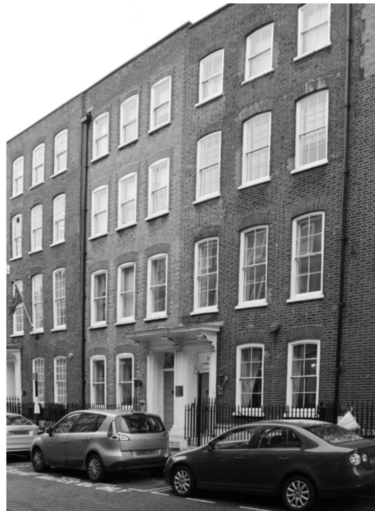
FIG 22. 2013 PHOTOGRAPH OF FRONT ELEVATIONS TO NOS. 14 AND 15 (REFER TO FIG.18 1965 PHOTOGRAPH)
