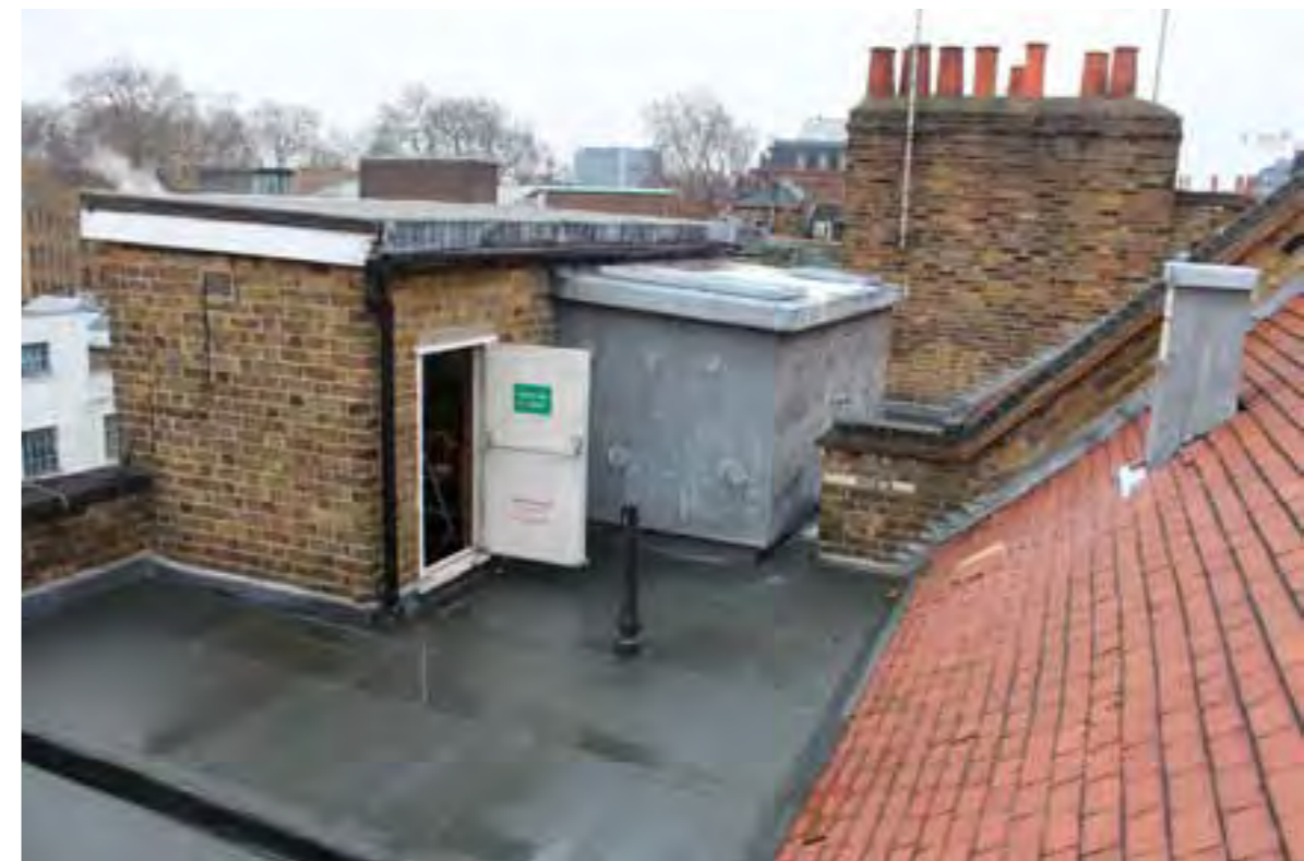
FIG 32. POST-1964 MAIN ROOF EXTENSION AND LIFT MOTOR ROOM TO NOS. 14 AND 15
