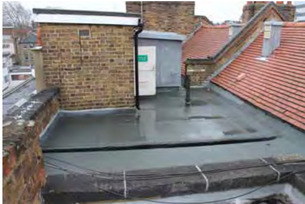
FIG 33. POST-1964 MAIN ROOF EXTENSION
