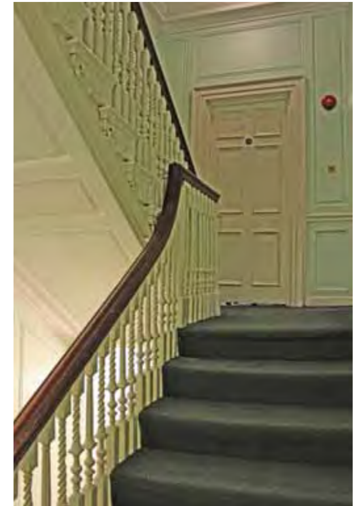
FIG 48. FIRST FLOOR STAIR AND LANDING AT NO.14
