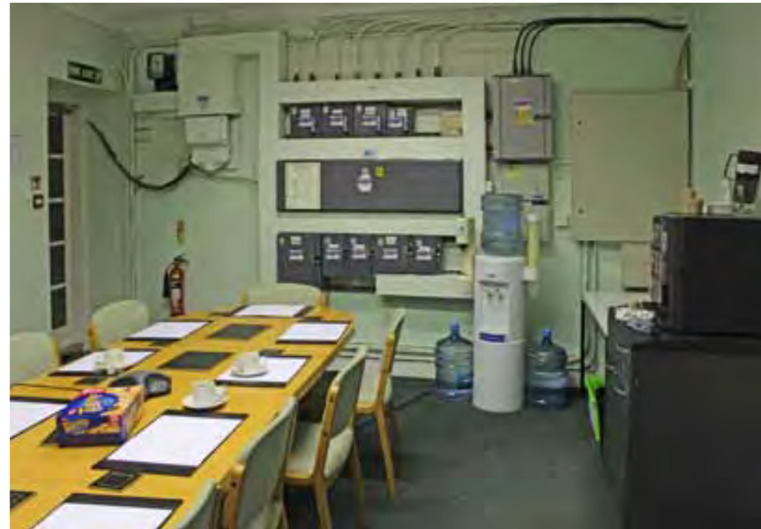
FIG 37. BASEMENT FRONT ROOM TO NO.14
