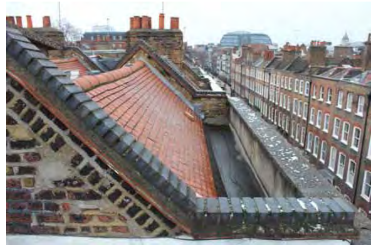
FIG 31. MAIN ROOF AND FRONT PARAPET GUTTER TO NOS.14 AND 15
