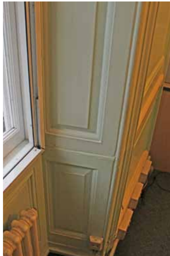
FIG 46. FIRST FLOOR FRONT ROOM SHUTTERS AT NO.14
