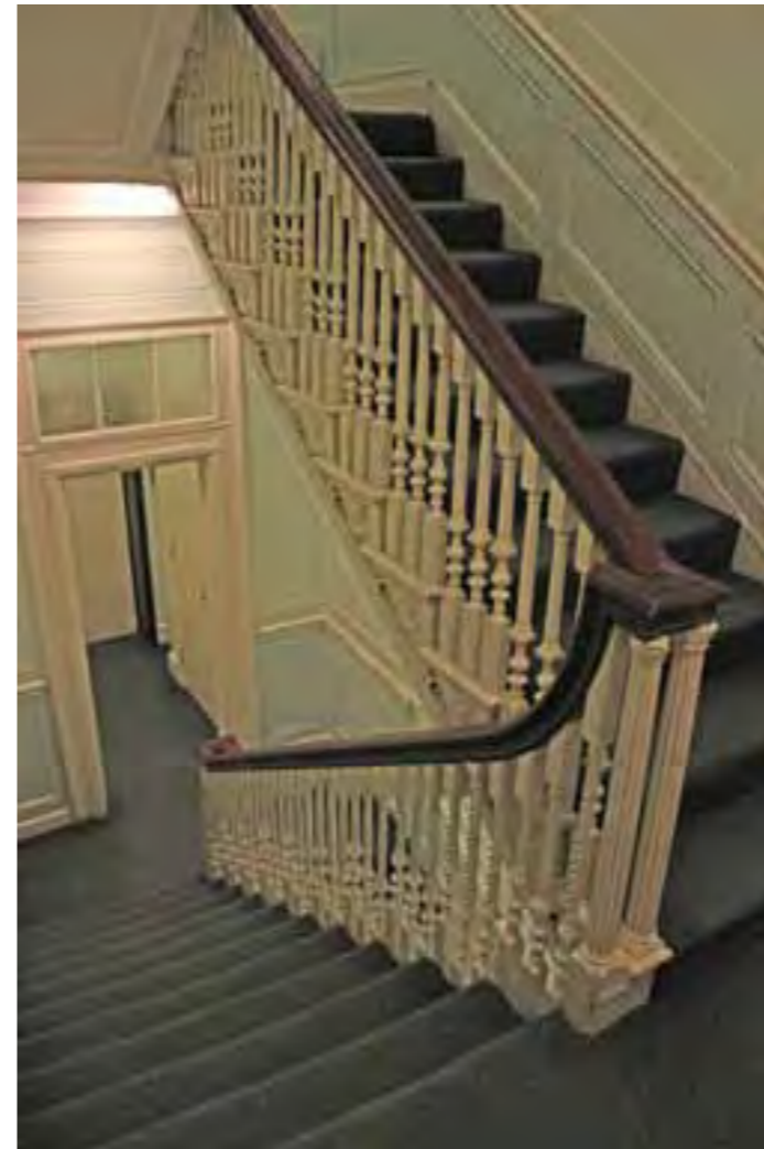
FIG 52. SECOND FLOOR STAIR AND PANELLING AT NO.14
