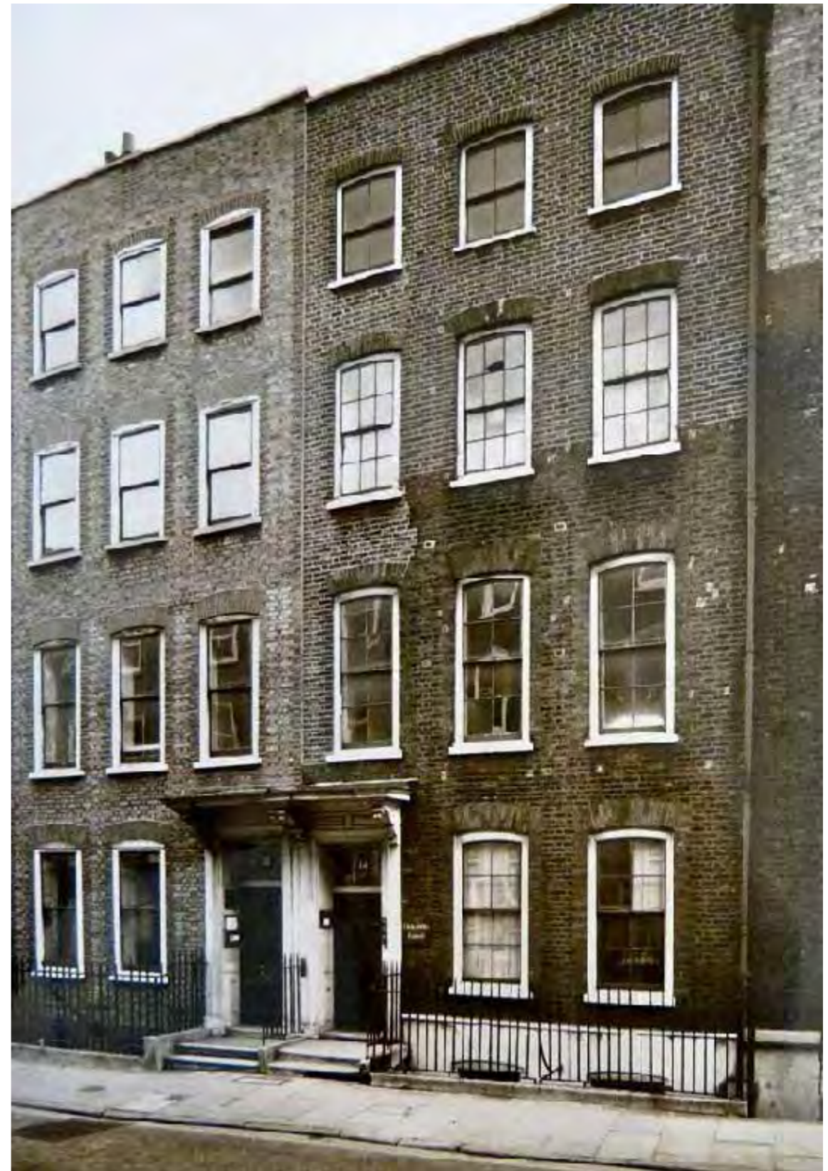
FIG 18. 1965 PHOTOGRAPH OF THE FRONT ELEVATIONS OF NOS. 14 AND 15 GREAT JAMES STREET (SOURCE: CAMDEN TOWN HALL, PLANNING DEPARTMENT)
