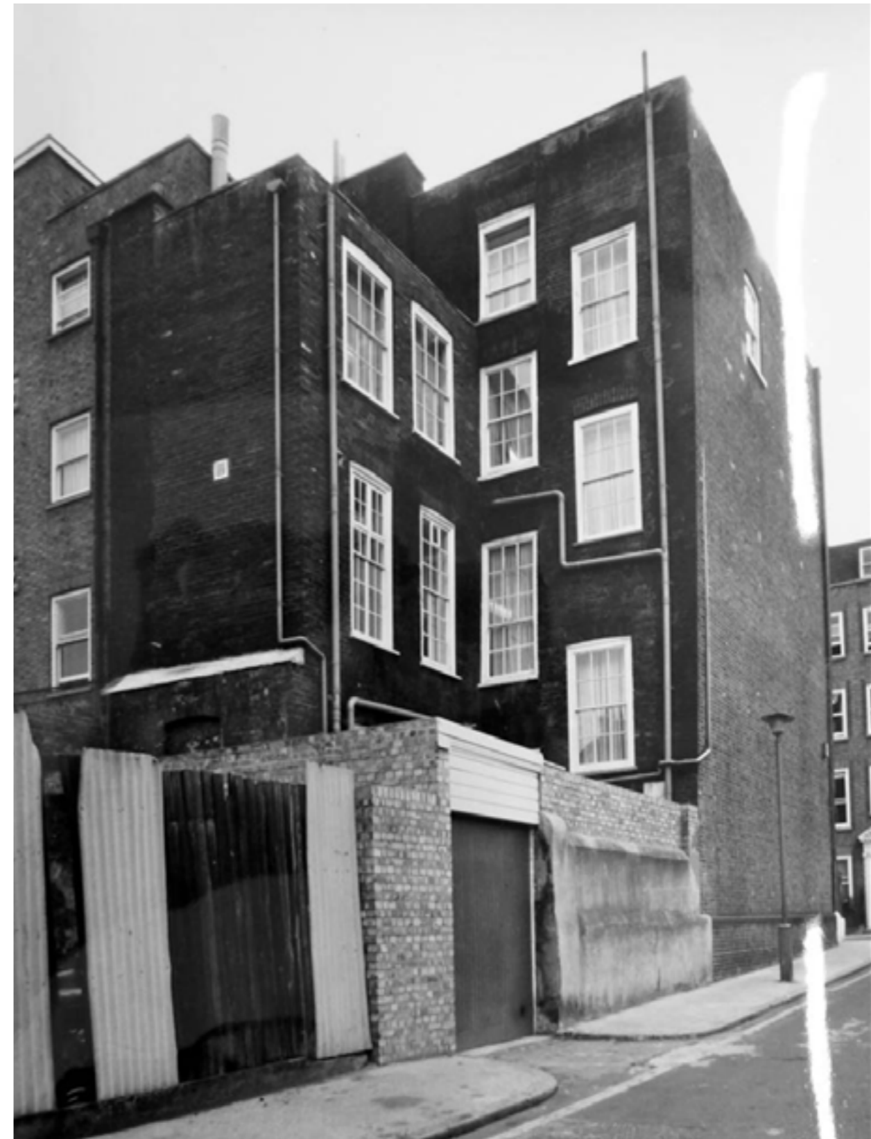
FIG 20. 1975 PHOTOGRAPH OF THE REAR ELEVATION OF NO. 16, SHOWING A SMALL PART OF NO.15 (SOURCE: LONDON METROPOLITAN ARCHIVES)
