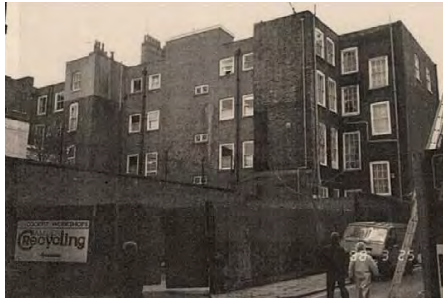
FIG 21. MARCH 1988 PHOTOGRAPH OF REAR ELEVATION OF NOS. 14 AND 15 GREAT JAMES STREET (SOURCE: ENGLISH HERITAGE PHOTOGRAPHY LIBRARY).
