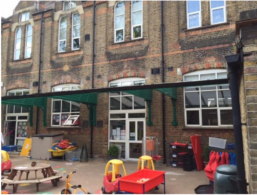
Photo 1: The canopy as constructed.
