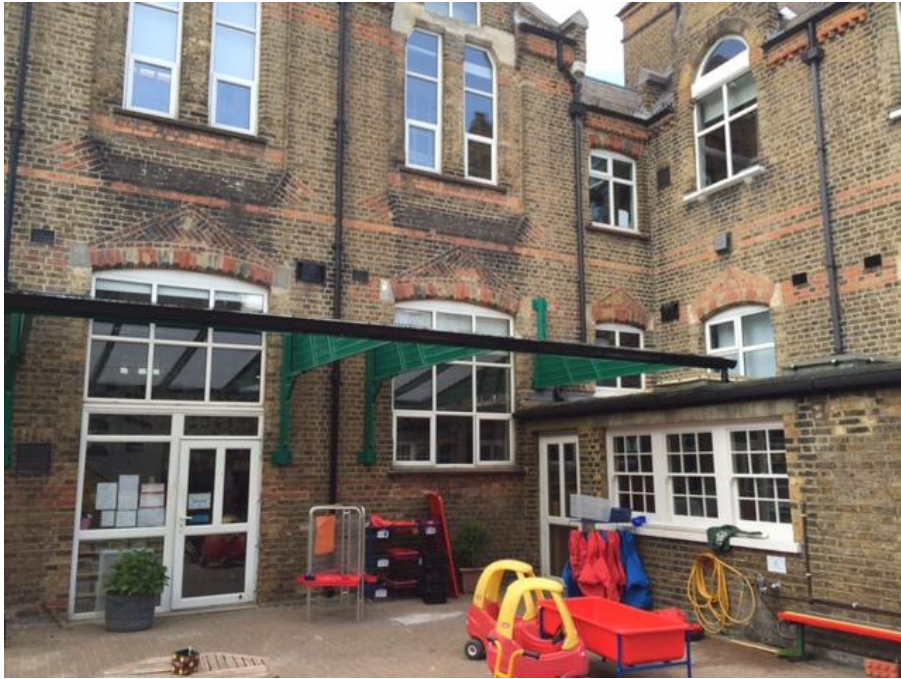
Photo 3: The canopy as constructed.
