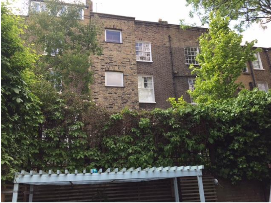
Photo 5: The rear of Gloucester Crescent.
