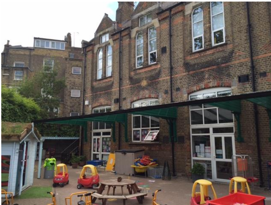
Photo 2: The canopy, looking towards the rear of Gloucester Crescent.
