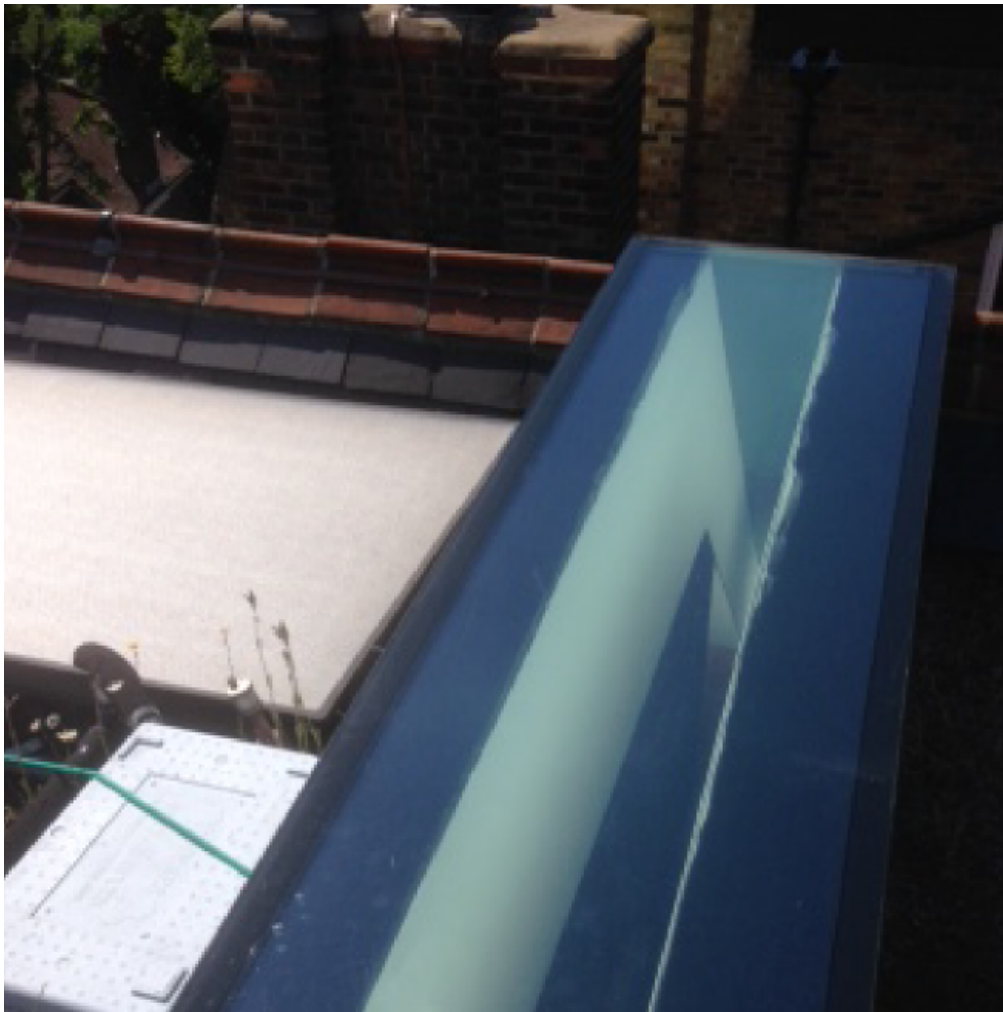
Photo 7: Central flat roof area – rooflight and solar panel
