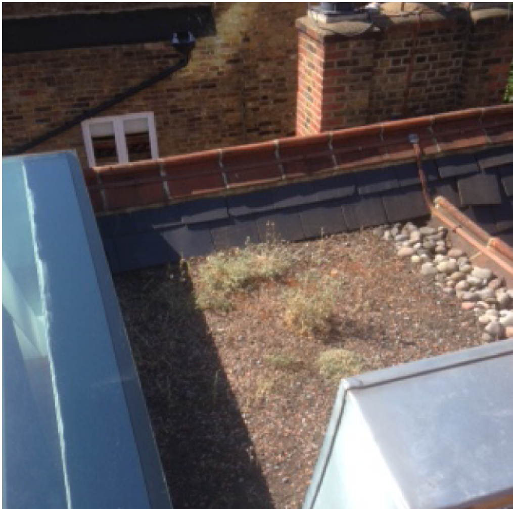
Photo 9: Central flat roof area – brown roof, rooflight and air conditioning unit
