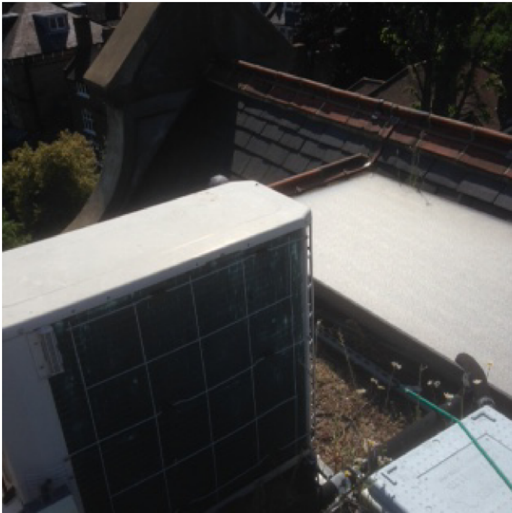
Photo 6: Central flat roof area – air conditioning units and solar panel
