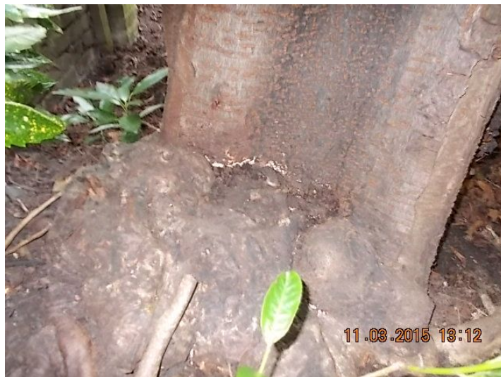
Photograph 3: Decay on T19
