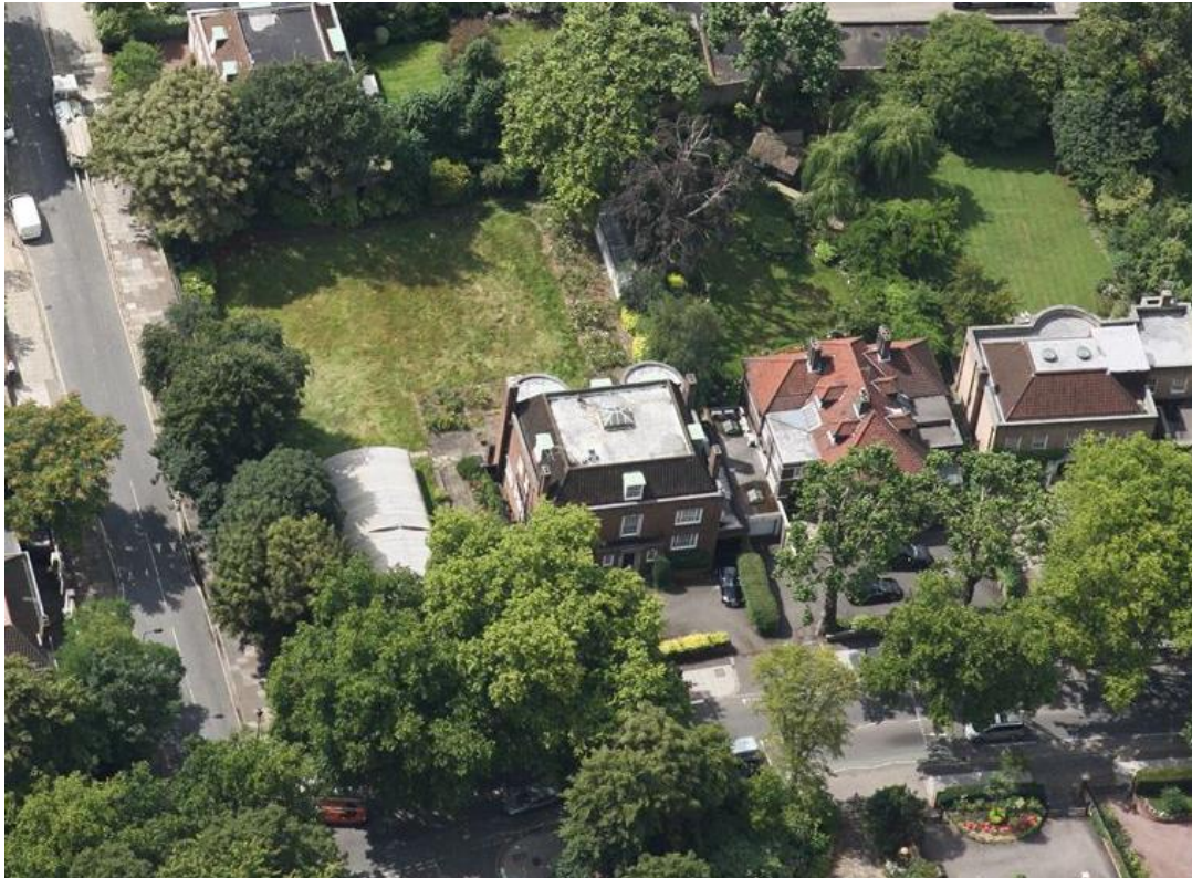
Above: View to the front of 73 – 75 Avenue Road
