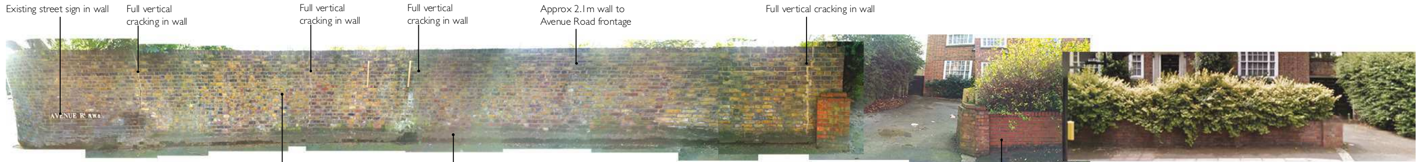
Fig. 17 Existing Avenue Road Boundary Wall
