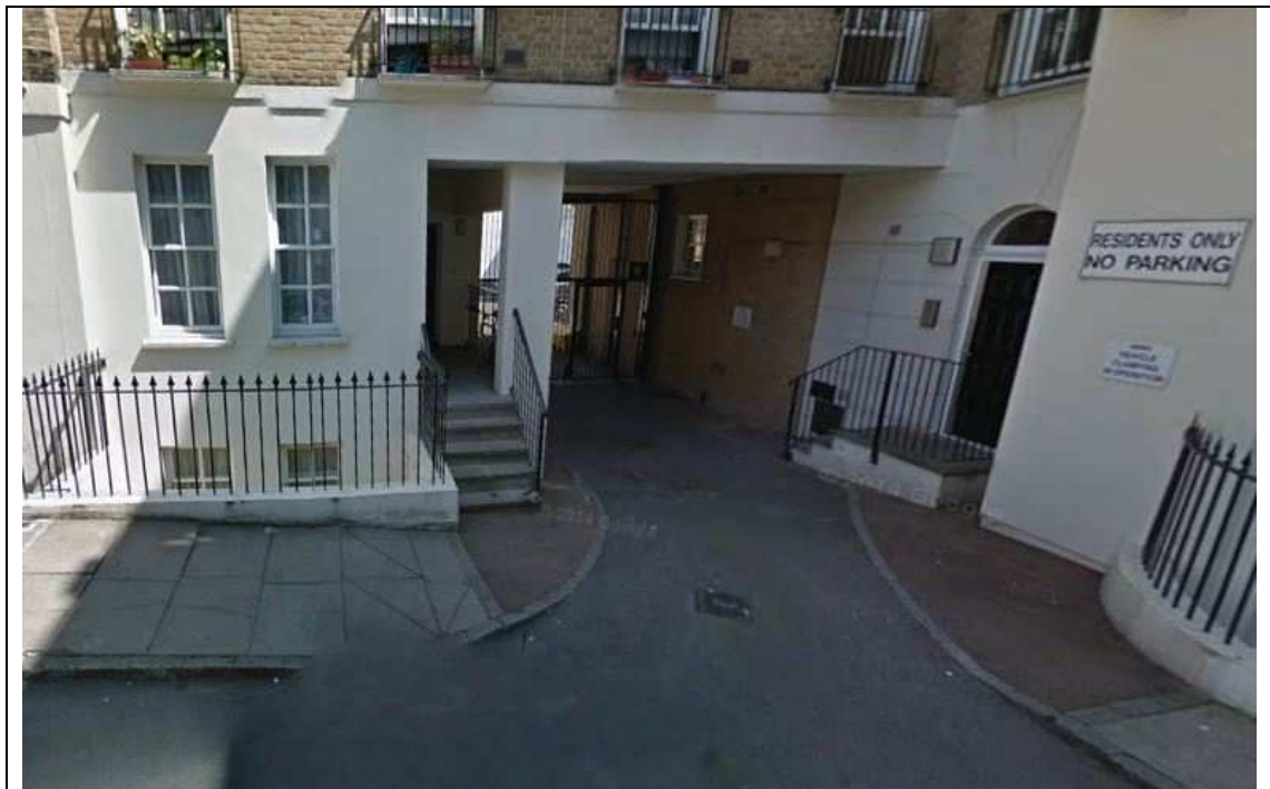
Figure 2 Covered passageway from Burton Street leading to rear car park, showing narrow access, proximity of pedestrian entrances and orientation relative to the road
