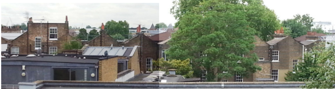
View of 51-61 Rochester Place from north
