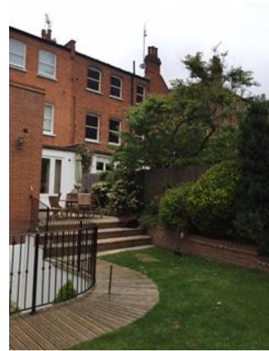
View from rear of No 2
