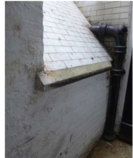
Concrete 'drip' proposed to be removed to facilitate installation of proposed lift. The majority of this area as seen will remain intact and only covered by the proposed lift construction.
