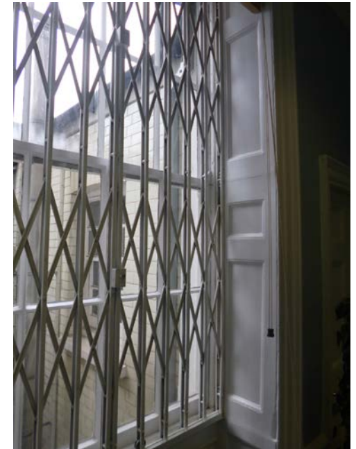
Existing window shutters and structural opening maintained - security bars and 1930's sashes proposed to be removed
