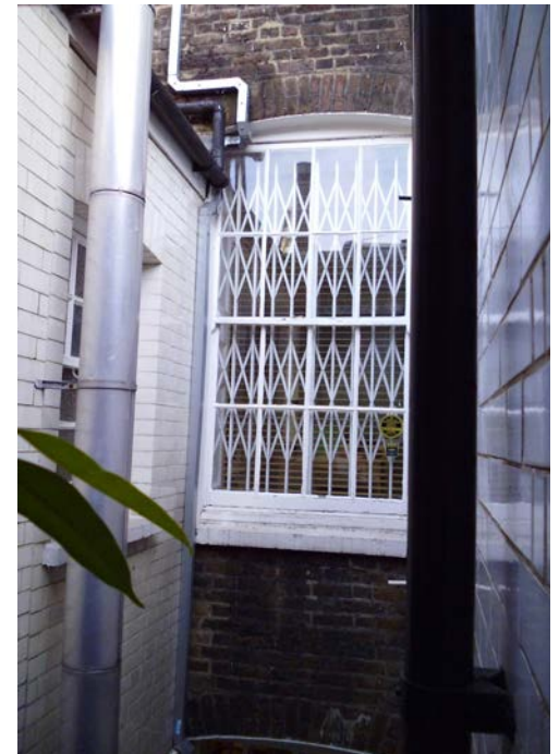
Existing rear window at ground level retained as an opening; existing sashes removed with boxes retained.
