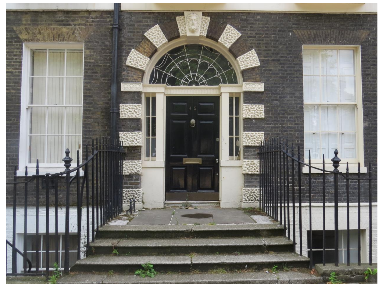
Fig. 4. Photograph showing the main entrance to 42 Bedford Square, with opportunity for enhancement by replacing existing concrete steps in stone to match adjacent properties.
