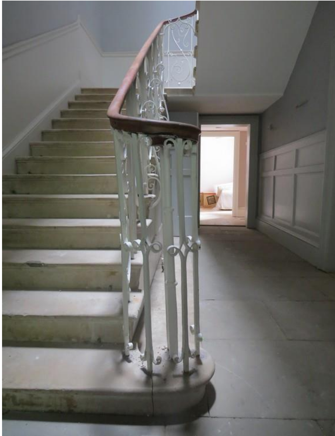
Fig. 5. The principal staircase where it begins at the ground floor level.
