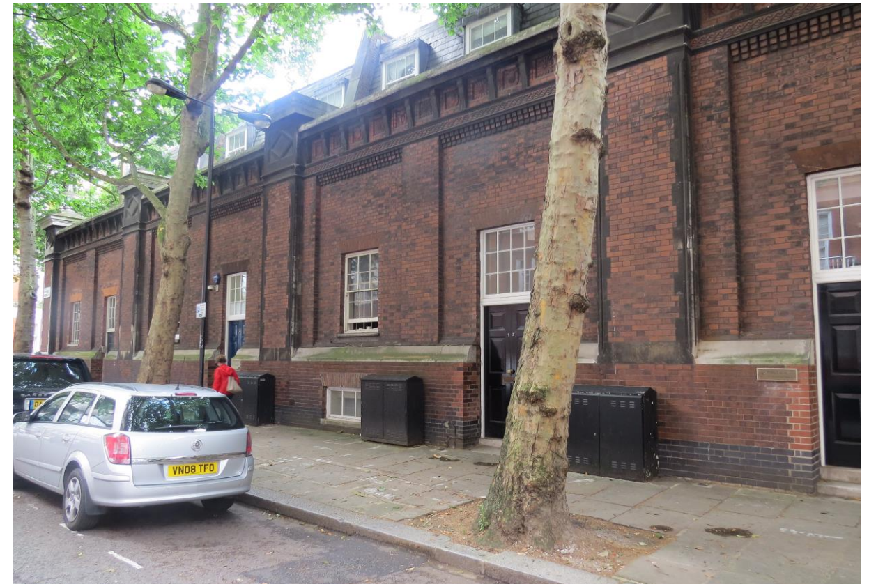
Fig. 11. View of the mews building facing Bedford Avenue, which was developed in the Edwardian period and lined with mature London Plane trees.
