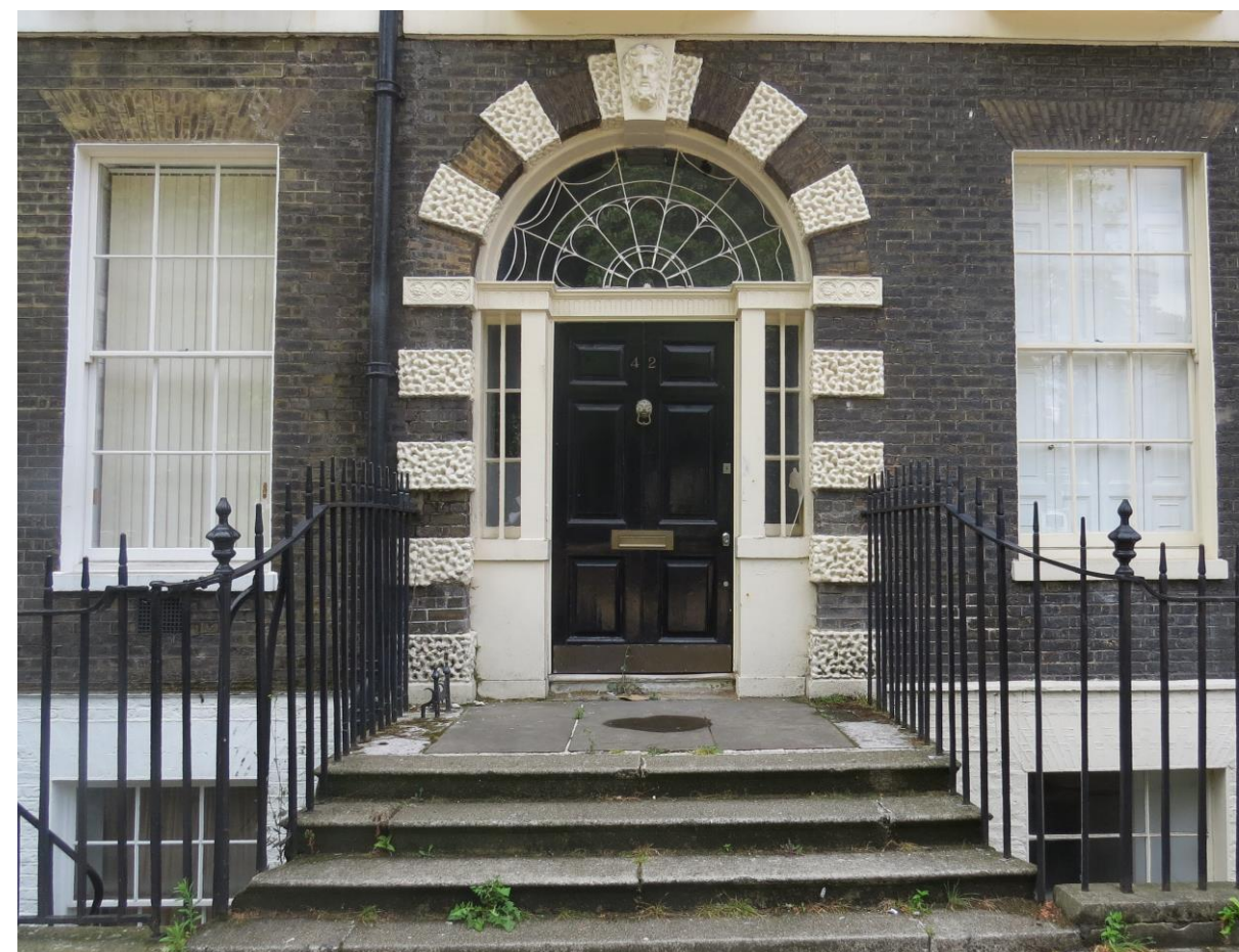
Fig. 4. Photograph showing the main entrance to 42 Bedford Square, with opportunity for enhancement by replacing existing concrete steps in stone to match adjacent properties.
