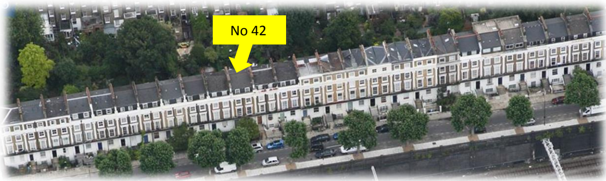
Fig 2: Mornington Terrace – listed row – Nos 26 - 52
