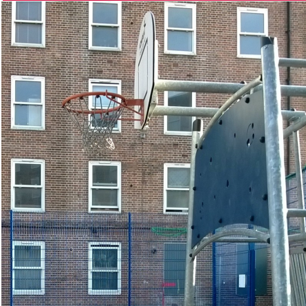
Demolition of Block Q and Reduction of Basket Ball Court
