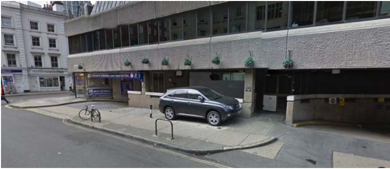
Existing entrance ramps
