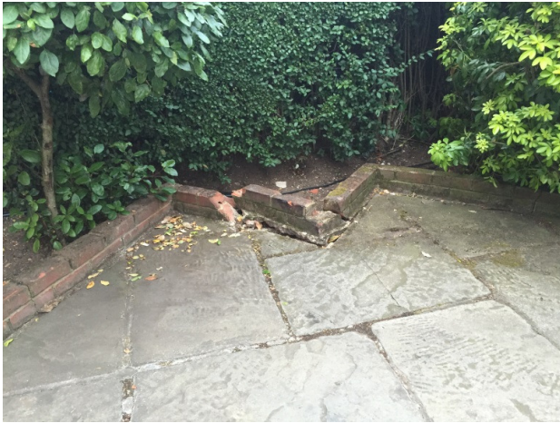
Photos 2 & 3: Damage to the flowerbed brick upstand due to the tree.
