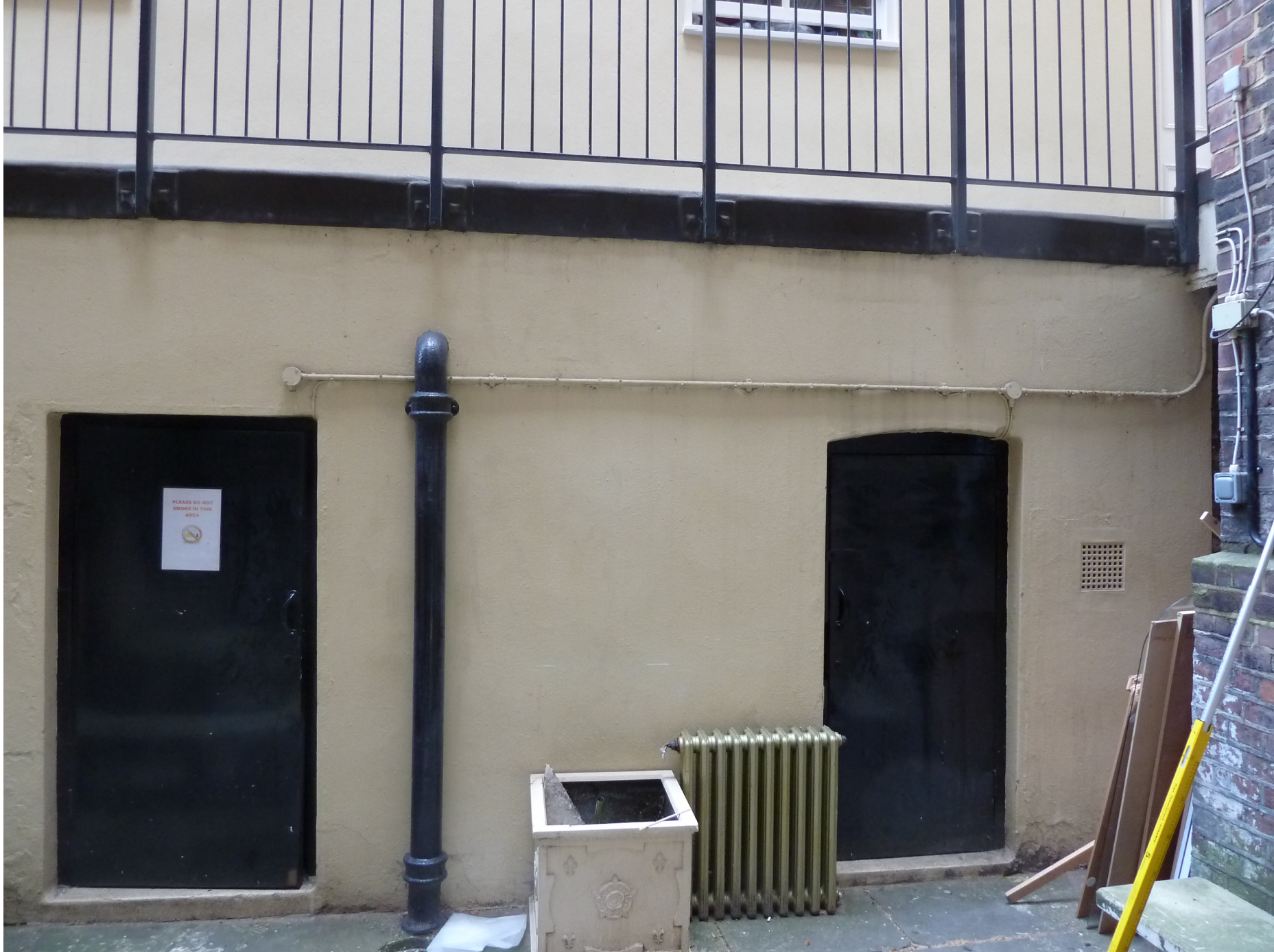
6. 99 Great Russell Street - Lower Ground Floor Vaults and Walkway
