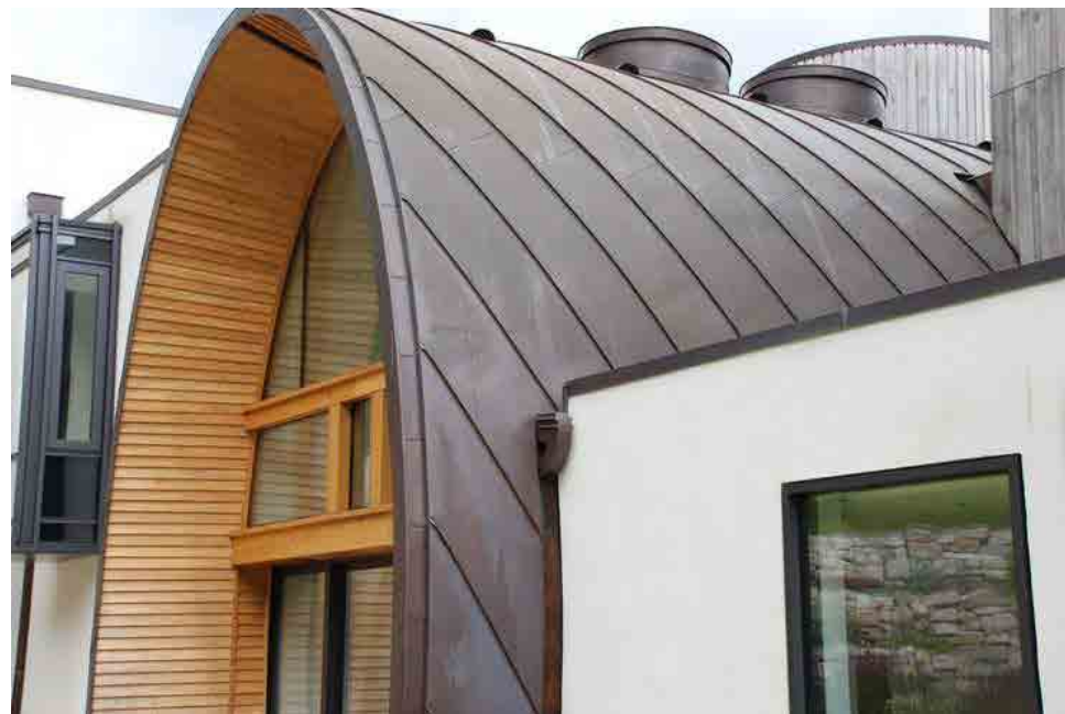
Fig 17 Zinc Cladded Roof
