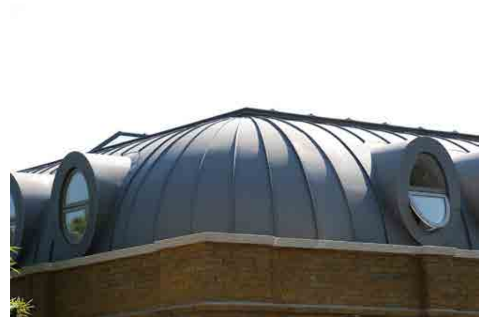
Fig 19 Zinc Mansard Roof
