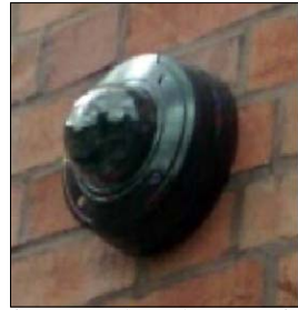
(10. image of specified camera)
