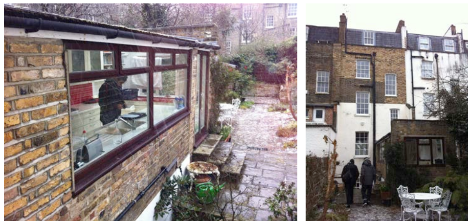
Existing extension and ground floor terrace:
