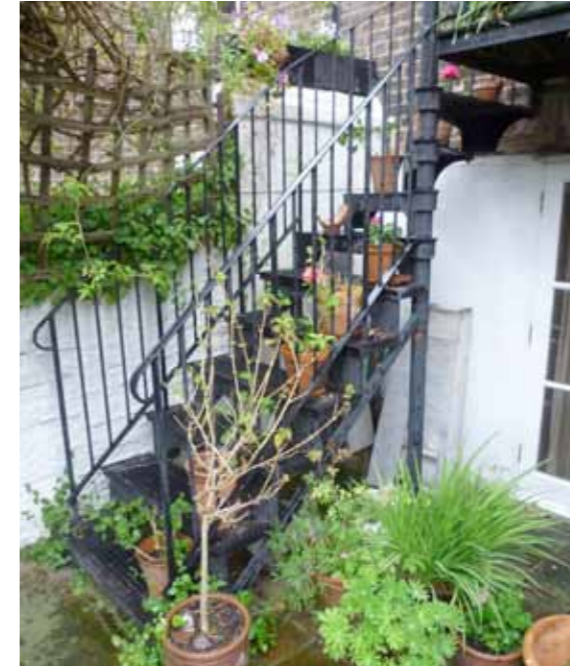
FIGURE 3.3: Existing rear staircase
