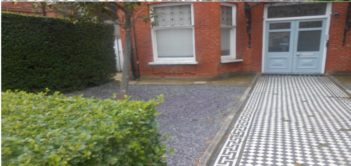
Top: Image of front of property, No.80 to the left (west), No.76 to the right (east)
