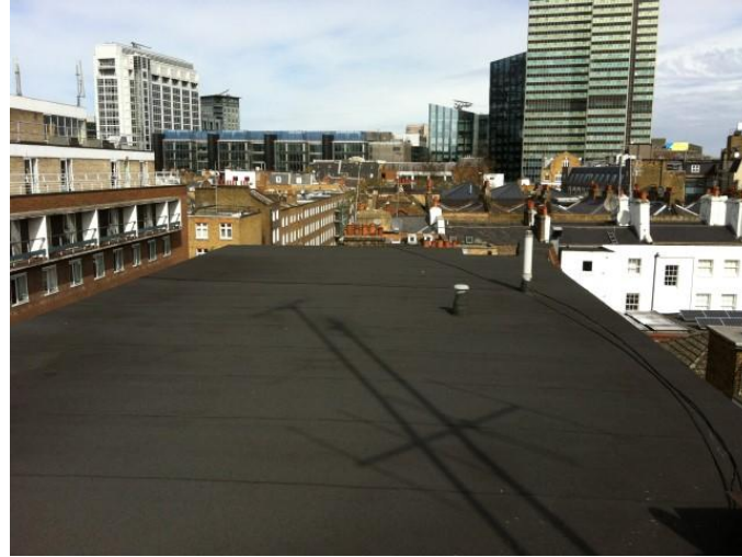
Exterior view of the flat roof.
