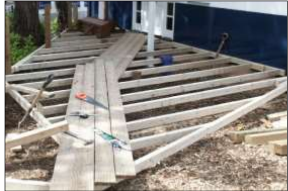
Photo 35: This deck supported above the ground on small posts provides a low-impact alternative to conventional stone patio surfacing in RPAs.
