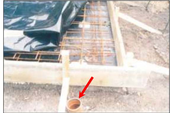
Photo 43: This reinforced base slab for a double garage has drainage provision (red arrow) beneath the structure to redirect roof runoff to supply roots with water.
