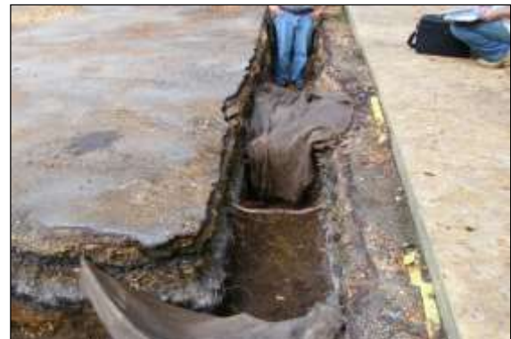
Photo 18: Exposed roots must be protected from light, drying out and extremes of temperature by covering with hessian sacking and boards until they can be covered back with soil.
