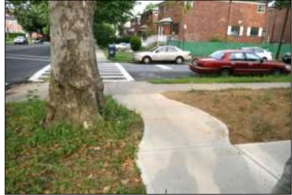
Photo 29: In some situations, it may be appropriate to cast a free floating concrete surface directly onto the soil surface provided provision is made to prevent soil contamination while the concrete is being poured, i.e. an impermeable membrane separating the concrete from the soil.
