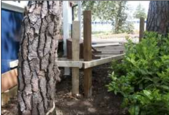
Photo 32: New surfacing can be supported above the ground on posts leaving the soil surface beneath undisturbed.
