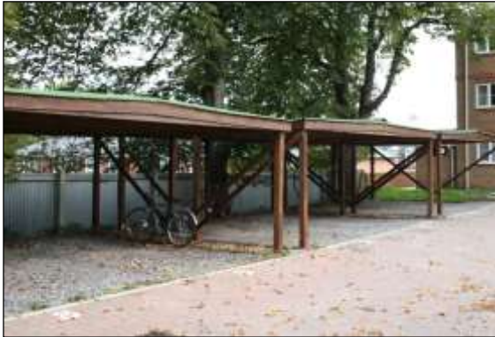
Photo 34: These carports are formed by wooden posts above a three dimensional cellular no-dig and load-spreading surface of permeable crushed stone.
