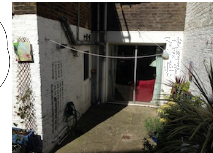
Photo 3 of existing rear elevaton
