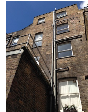
Photo 1 of existing rear elevaton
