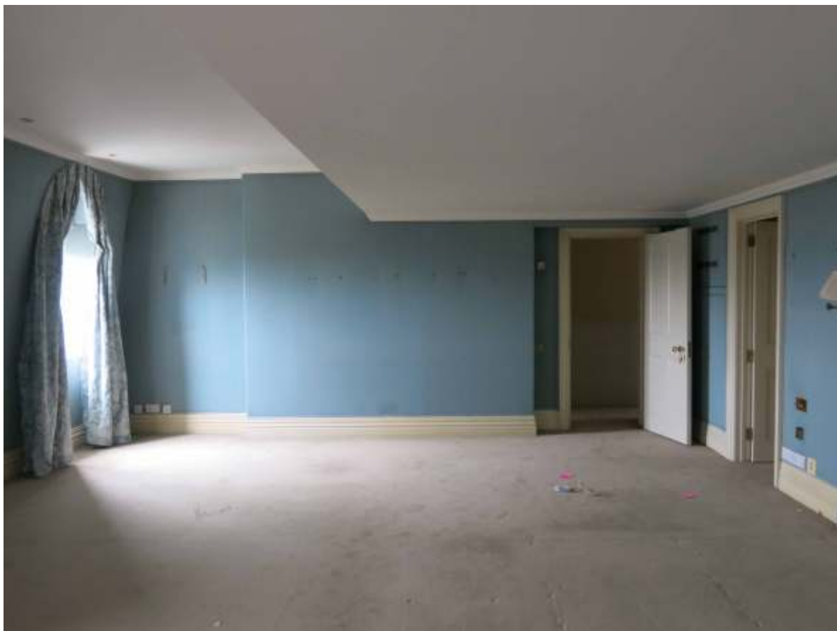
5.11: 4th Floor bedroom within No.6. Note the lowered ceiling attributed to the 1994 creation of an attic storey.
