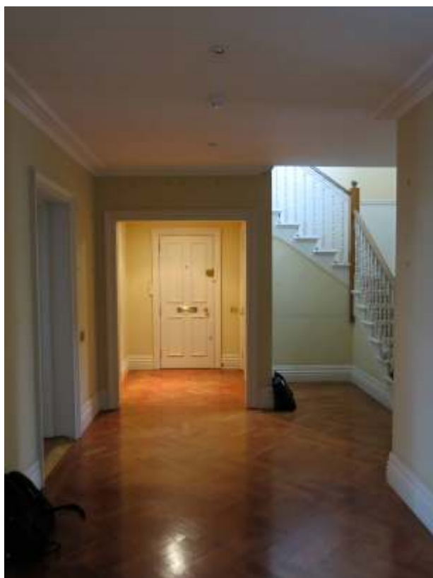
5.2: Entrance hall spanning No.6 & 7 with wall on left hand side the former external rear wall of the houses.
