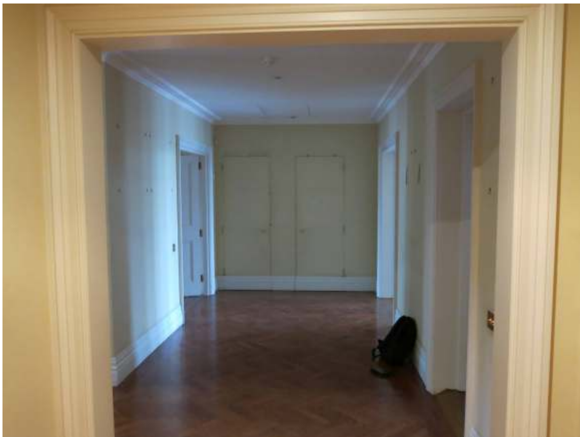
5.1: Entrance hall spanning No.6 & 7 with wall on right hand side the former external rear wall of the houses.
