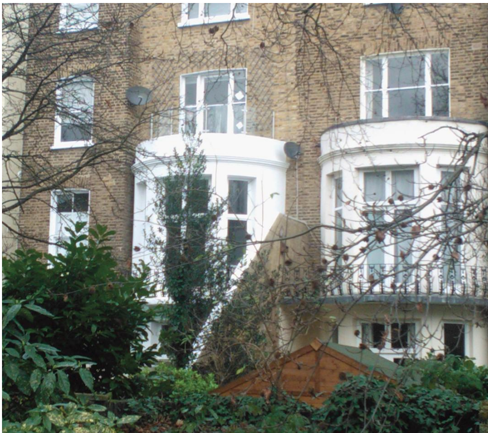
View of Units to rear of application site
