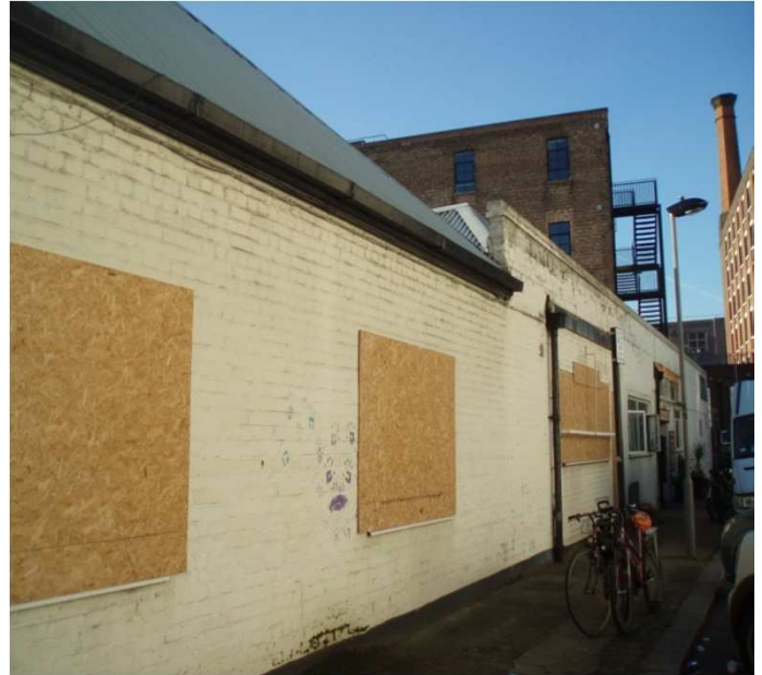
Image 10: Front of Disused Section of Greenwood Place
