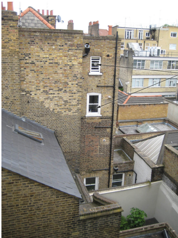
Kitchen windows to flats at 15 Rugby Street
