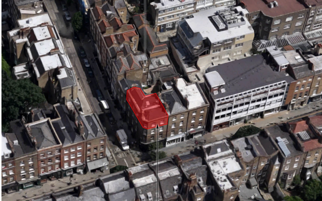
Flat 3, 52 Lamb's Conduit Street
