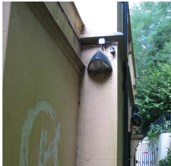
4 Light fitting, east elevation (prior to redecoration)
