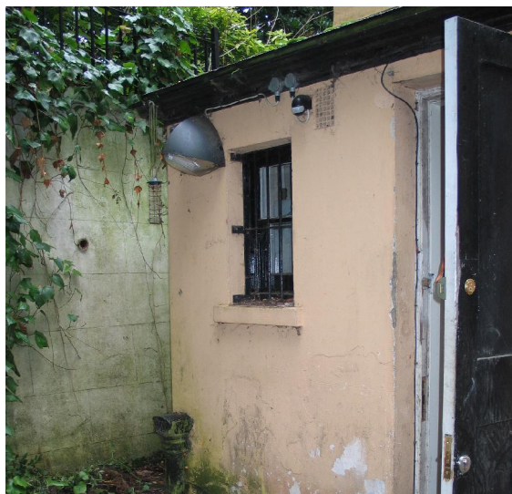
3 Part North elevation (prior to redecoration)
