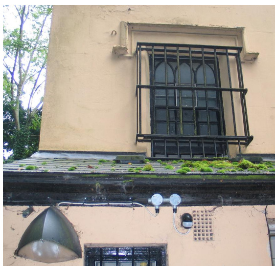
5 North elevation (prior to redecoration works)
