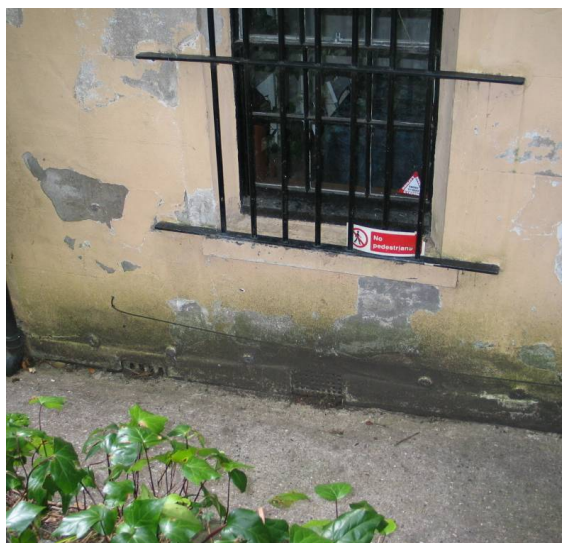
1 East elevation (prior to redecoration works)
