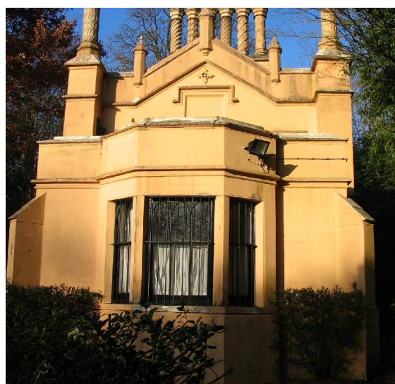
6 South elevation (prior to redecoration works)
