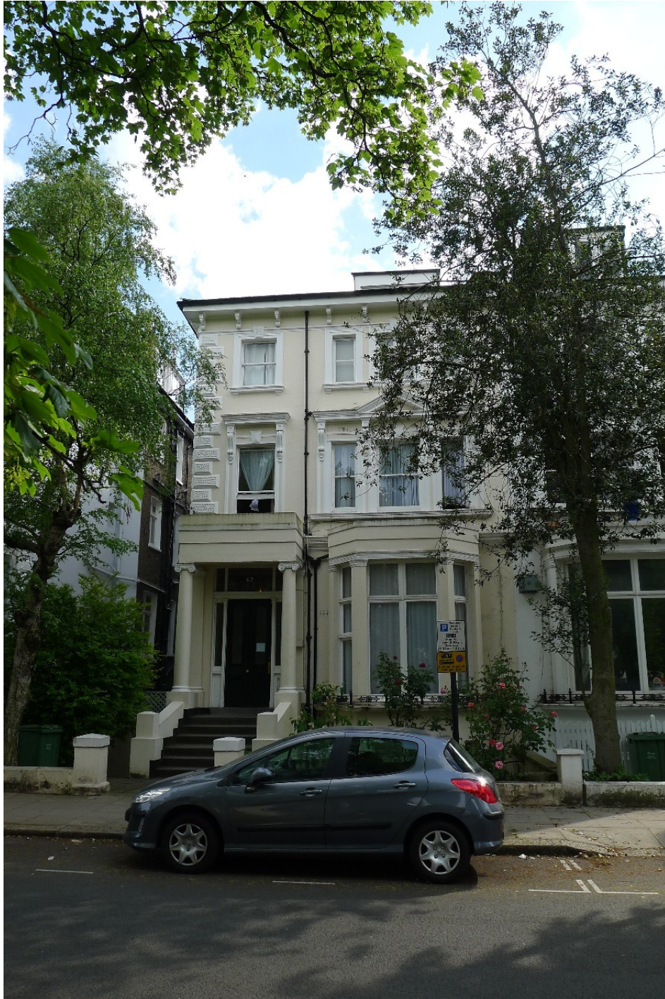
General view from Belsize Park Gardens
