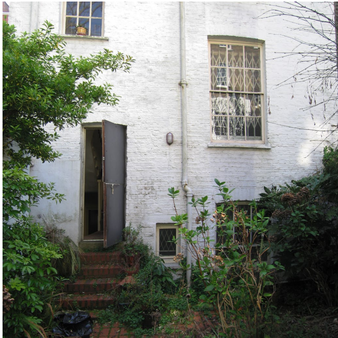
fig13. Current rear of 8 Thanet Street
