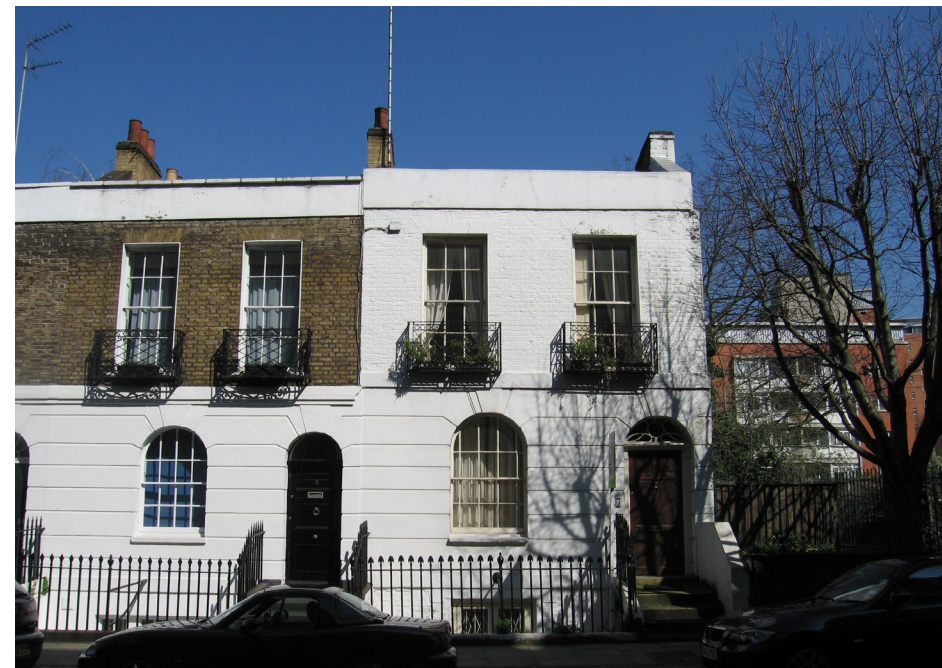
fig13. Current front of 8 Thanet Street
