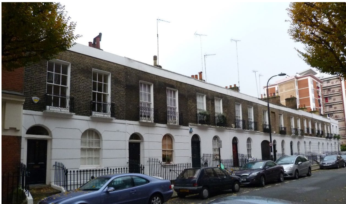
fig1. Current front of 8 Thanet Street
