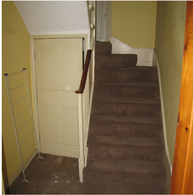
fig17. Staircase on lower ground floor
