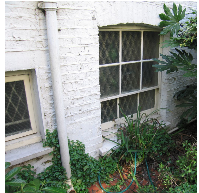
fig15. Rear lower ground floor window
