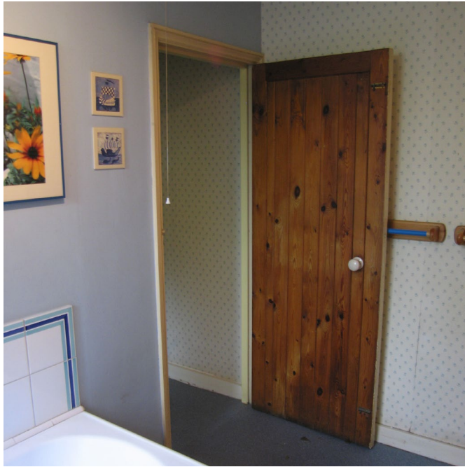
fig16. Door to lower ground floor bathroom
