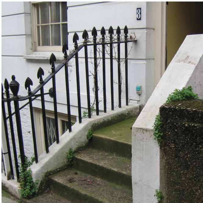
fig6. Iron railing at the front of 8 Thanet Street
