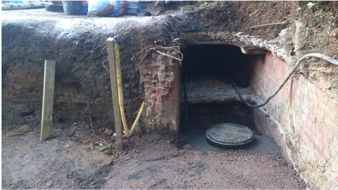
Photo 4 – Existing void exposed during site works to lay new services.
