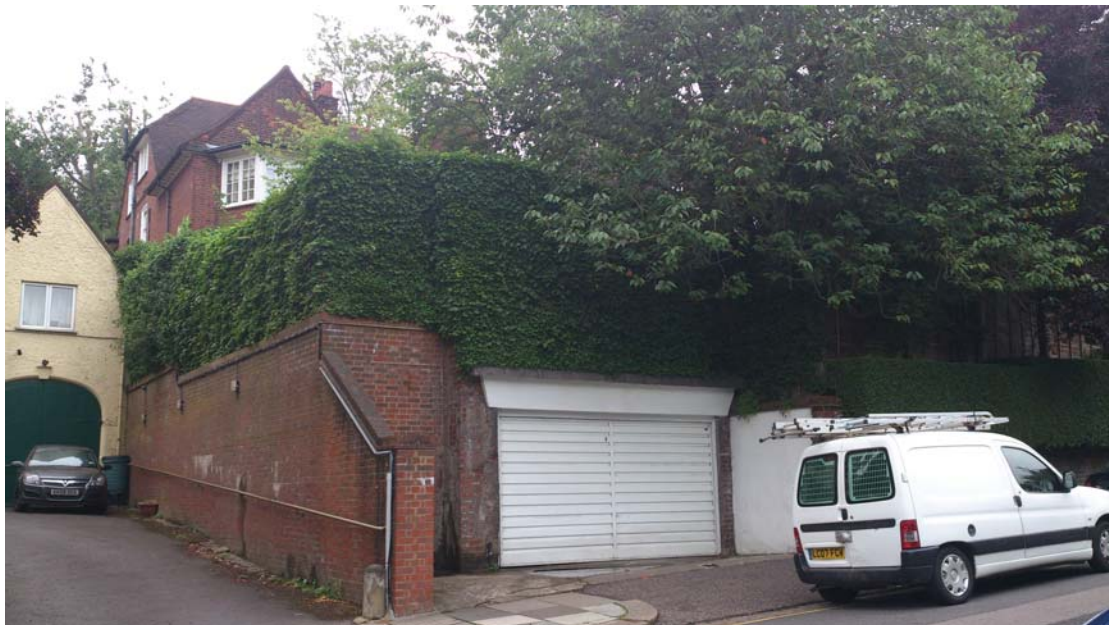
Photo 2 – Part front and side elevations taken from street (photo taken prior to the commencement of previously consented building works).
