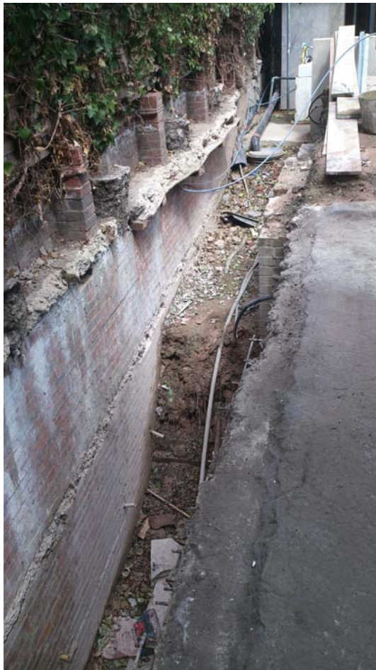
Photo's 5 & 6 – Existing void fully exposed.
