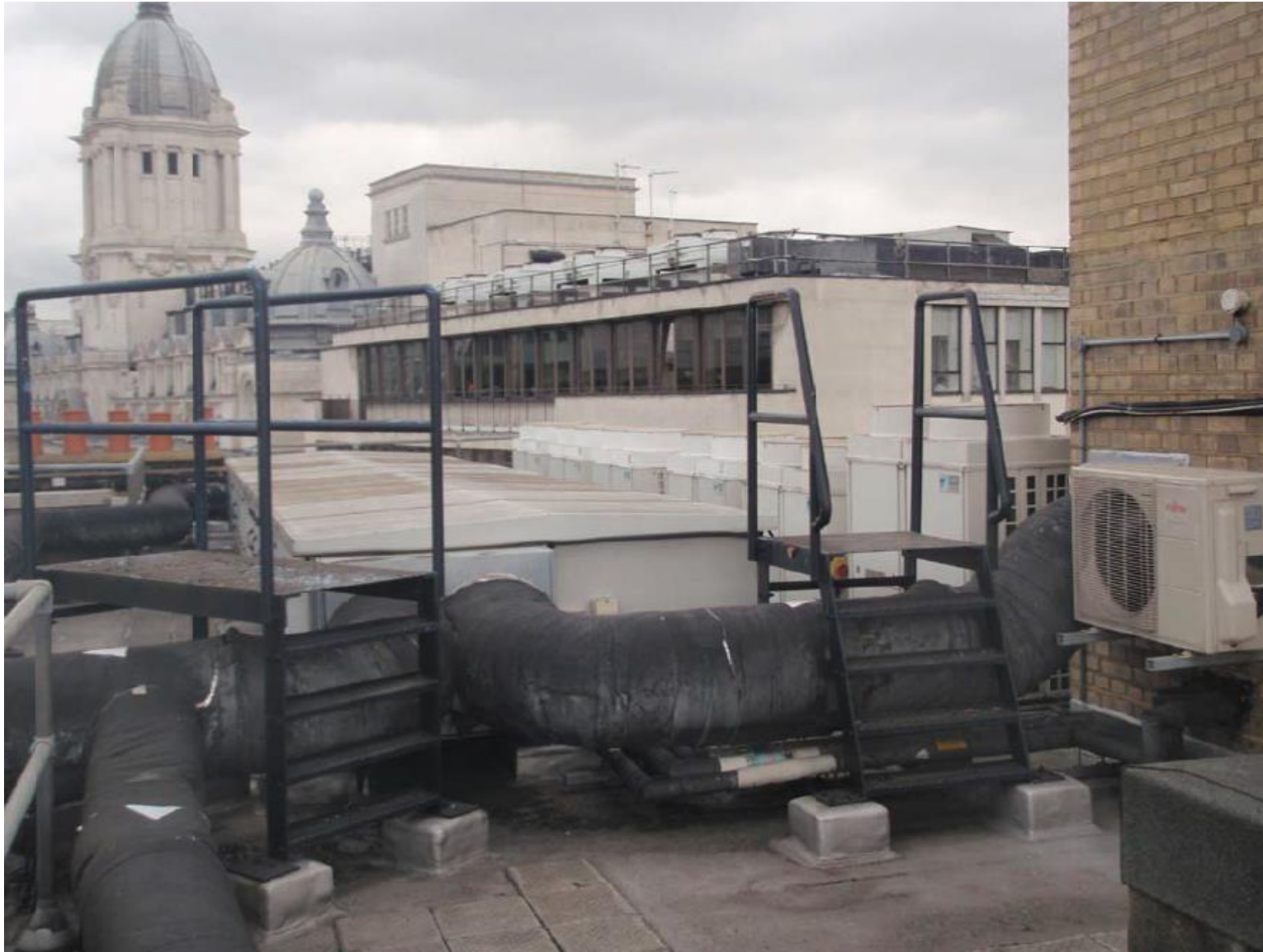
235 HIGH HOLBORN, LONDON WC1 Photograph of Existing Roof Installations
