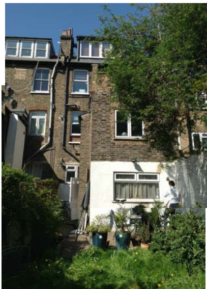
FIGURE 3: existing rear facade
