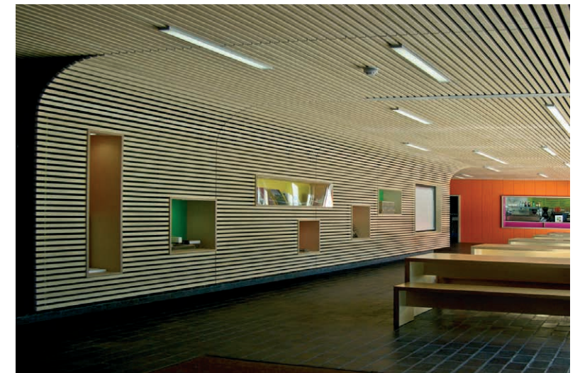
Timber batten linings to walls and ceilings to provide acoustic absorption
