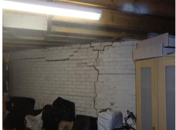
Fig 1.2 – Cracking in garage
