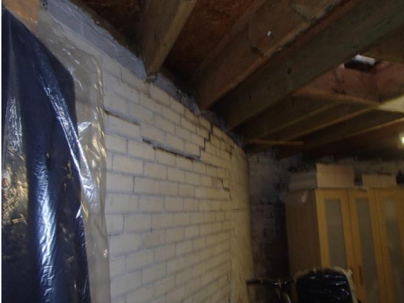
Fig 1.1 – Cracking in garage
