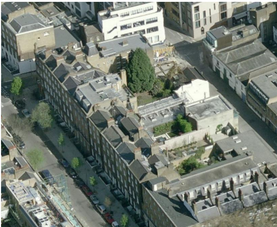
Picture 1 Site Location
