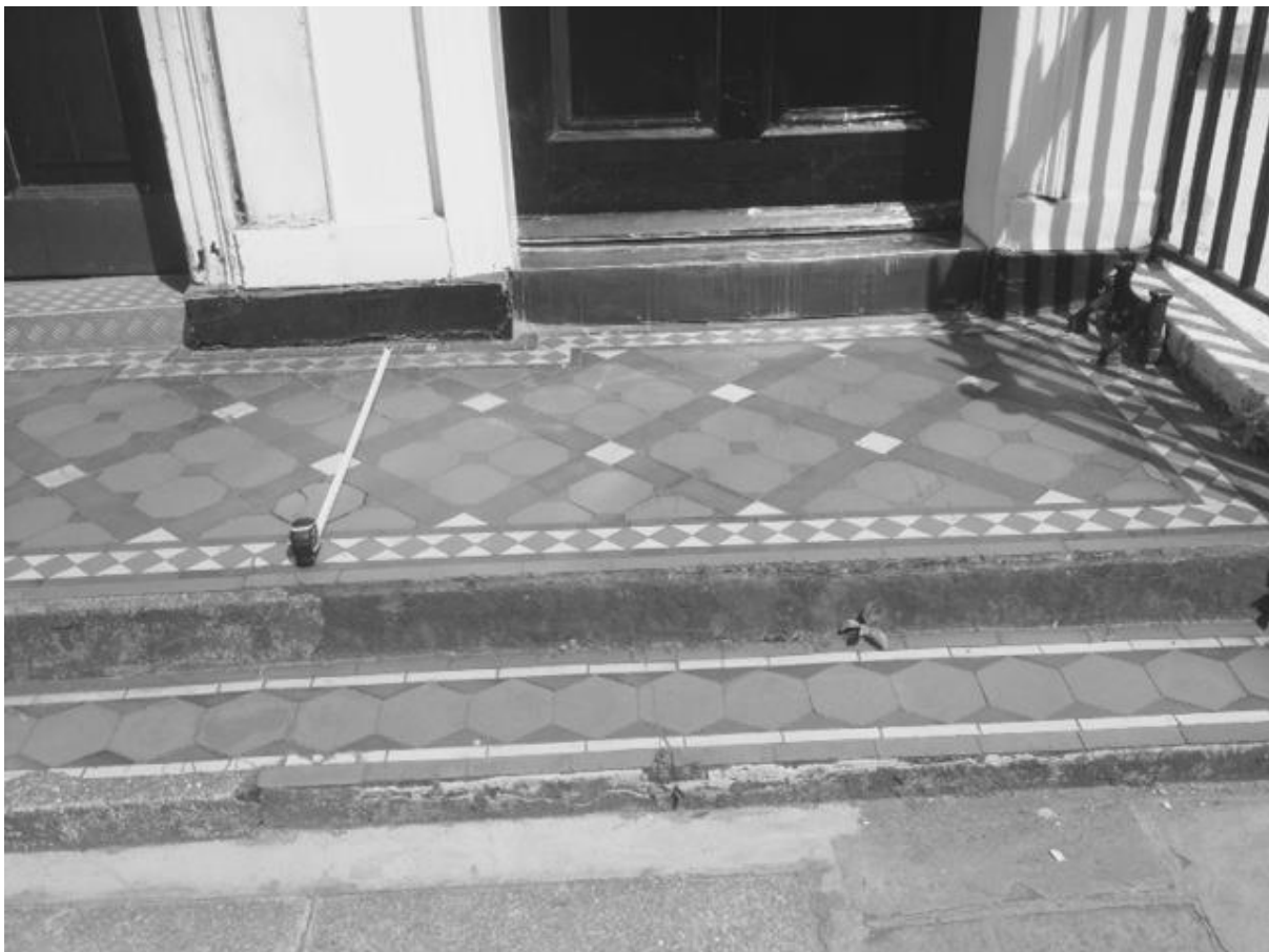
The tape measure represents the No8 side of the new plinth
