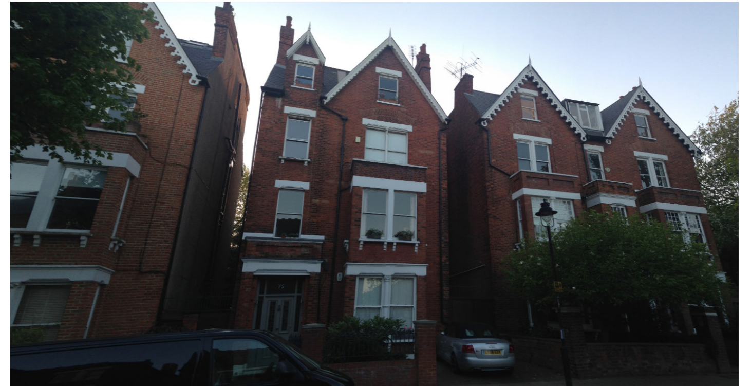
Proposed view from street showing enlarged rooflight at front. It would be largely hidden behind the two front gable dormers.
