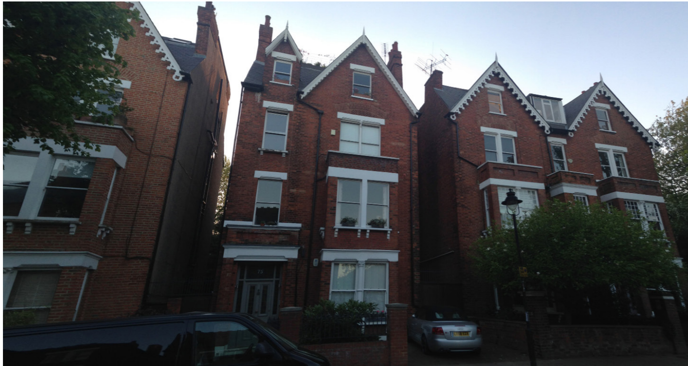
Existing view from street.
