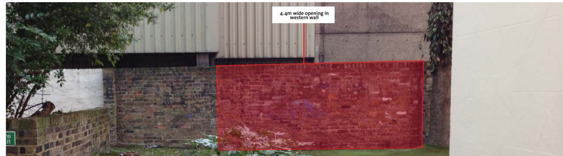
(2) 4.4m long section to be removed in western wall
