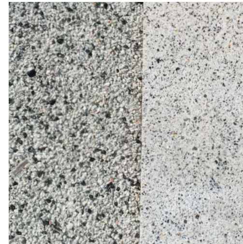
High quality concrete paving to replace Yorkstone
