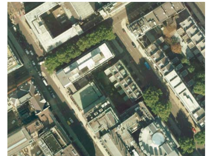
The existing tree framework to Endsleigh Gardens & Taviton Street
