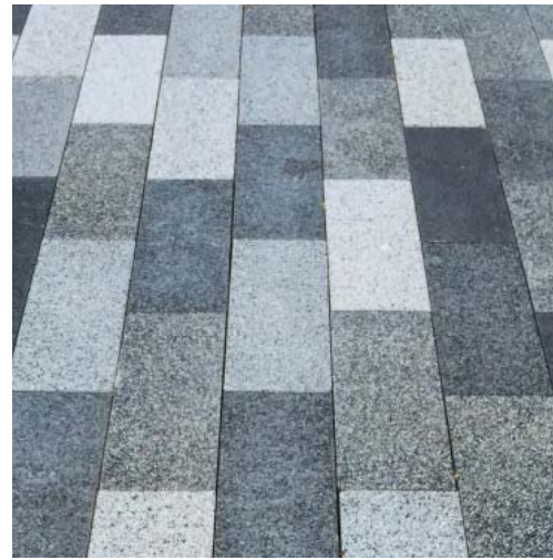
High quality concrete paving mix to route to cycle storage
