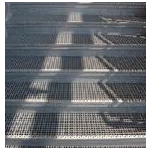
Access stairs from Taviton Street
