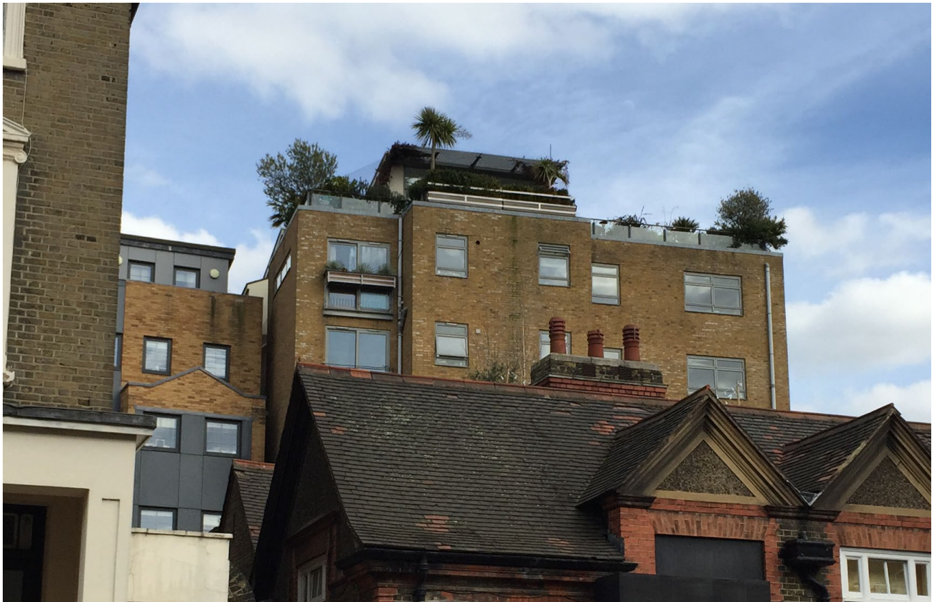
EXISTING VIEW FROM CLIFF VILLAS TO NORTH
