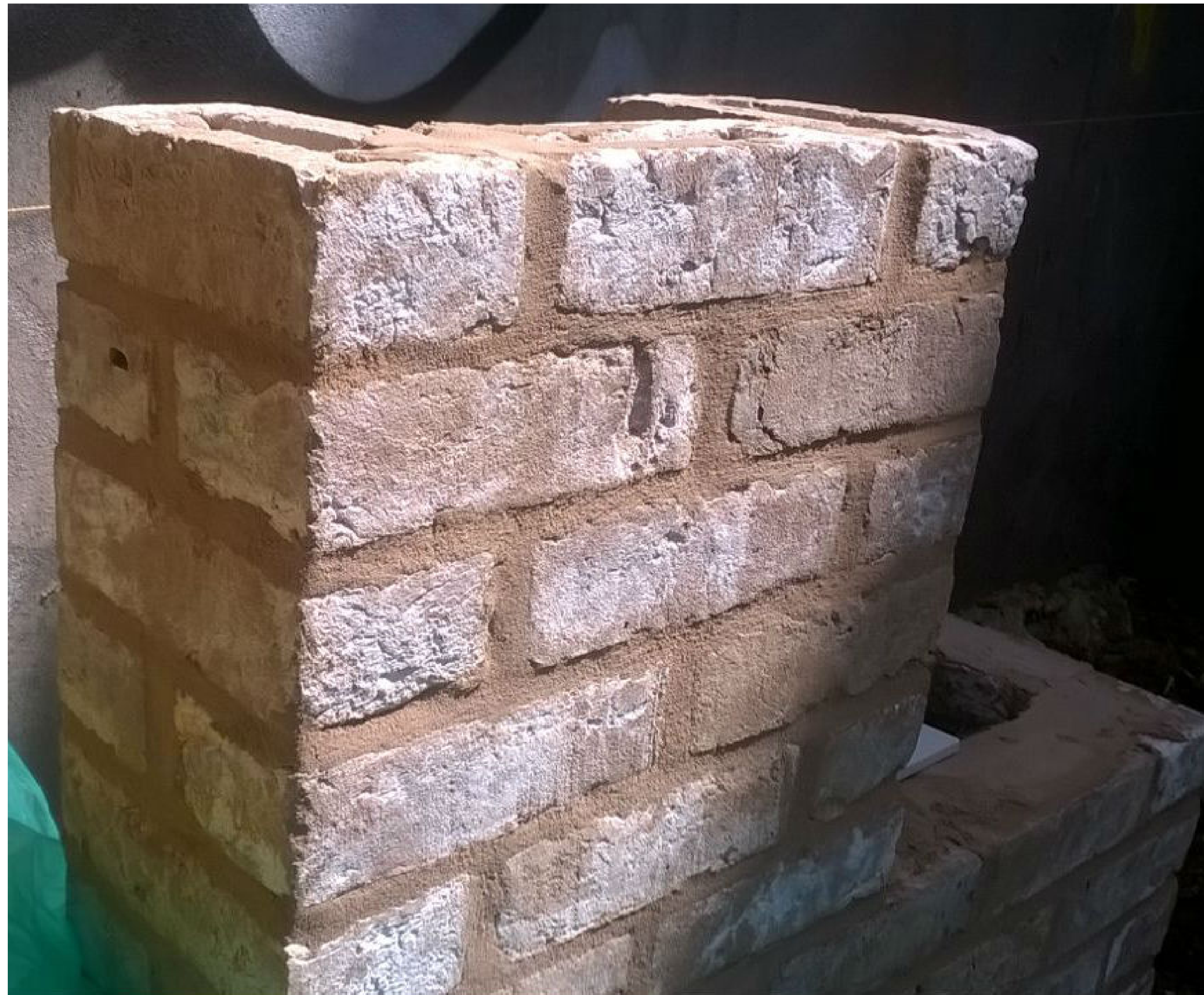
Brickwork panel showing brick colour, texture, mortar colour and joint finish
